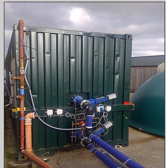
Fig. 3—Waste inlet / outlet, mixing lines and gas collection
