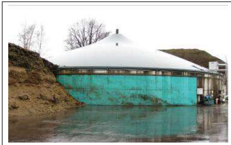
Figure 5 – Digestate storage tank for waste treatment plant with adjacent maize silage for energy crop plant
