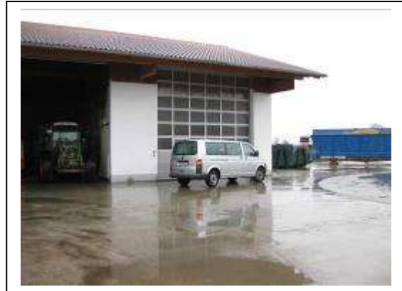
Figure 2 – Waste reception building that can be used to receive solid wastes (empty at time of visit)
