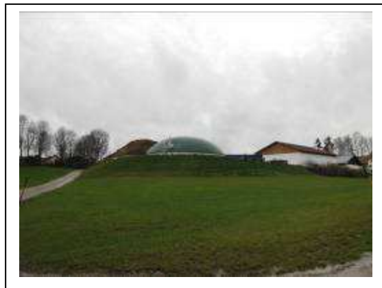
Fig 16 – The gas storage dome represents the only visible indication of the biogas plant from the public highway. The remainder of the plant has been landscaped to minimise visual impact
