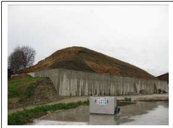
Figure 6 – Maize silage within clamp. Outer ring of primary digester with mixer service box in foreground
