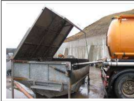
Figure 1 – Liquid greases being delivered to the hopper leading into the below ground reception tank
