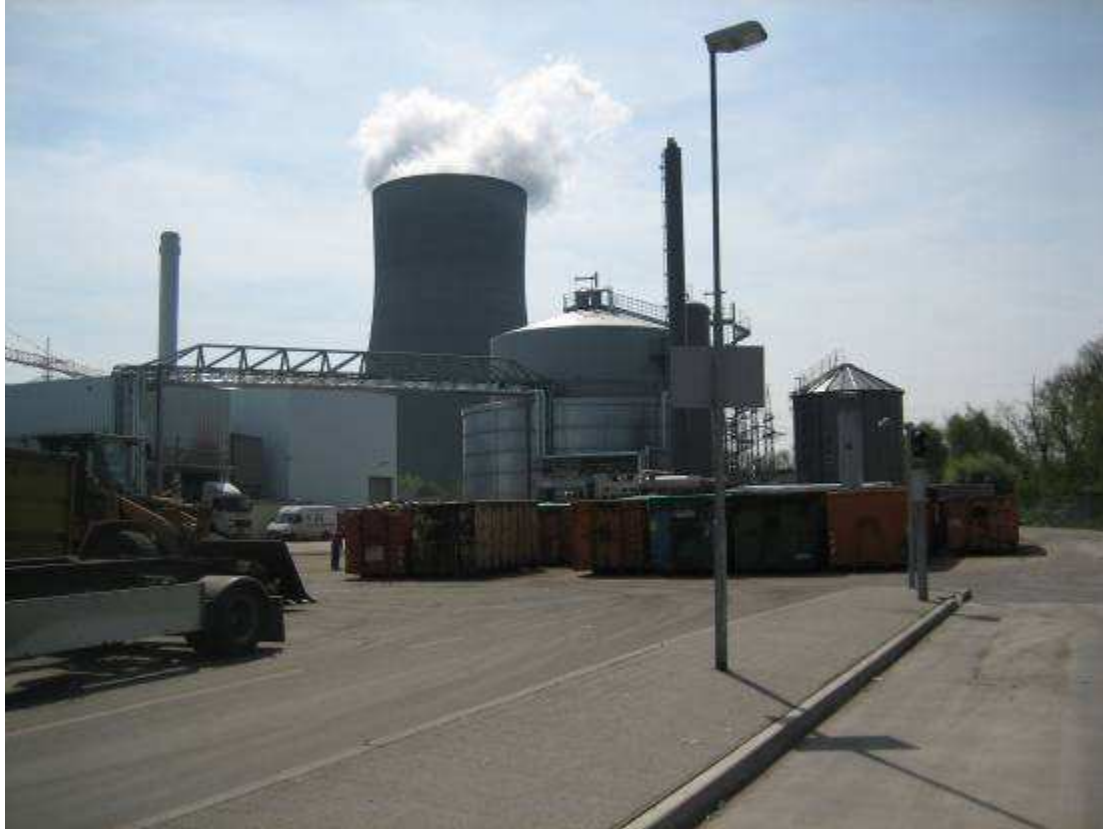
Figure 12 ISKA Plant at Heilbronn (power station in background)
