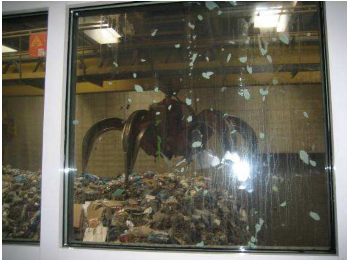
Figure 5 Wastes reception area (indoors) at Heilbronn
