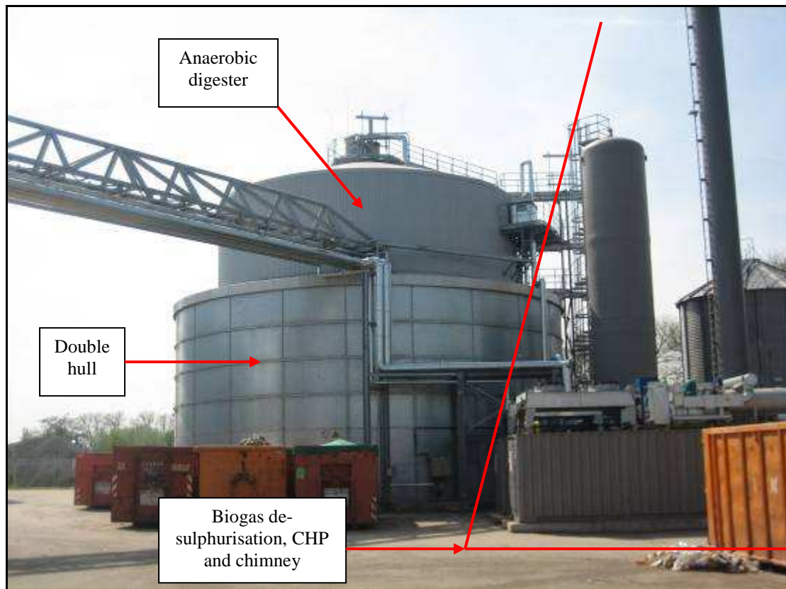
Figure 9 Anaerobic digester at Heilbronn
