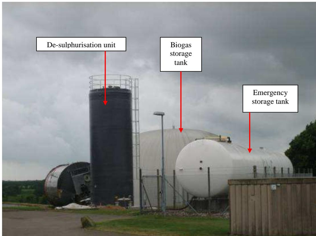
**Figure 7** Biogas buffer/storage tank, emergency storage tank and de-sulphurisation unit
