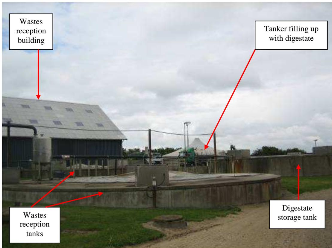
**Figure 6** Digestate storage tanks
