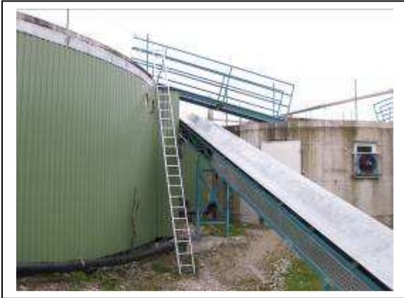
Figure 17 – Conveyer leading to one of two primary digesters (green). Adjacent concrete structure is the central control room housing pumping and heating manifolds and monitoring and control equipment.
