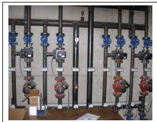
Figure 21 – Heating manifold located in central control room which distributes heated water to digesters.
