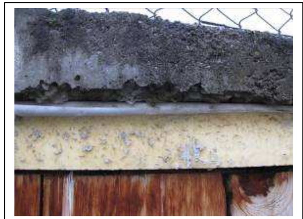
Figure 9 – Insulation to roof of secondary digester
