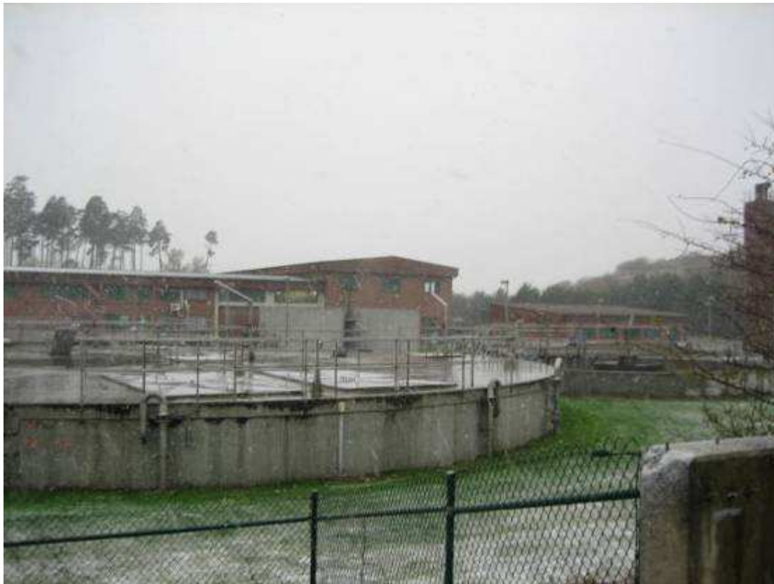
Figure 12 Wastewater treatment plant
