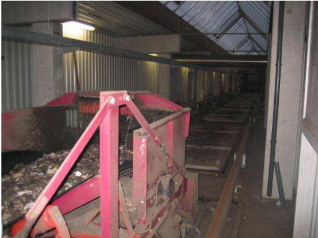
Figure 9 Waste entering tunnel composting system
