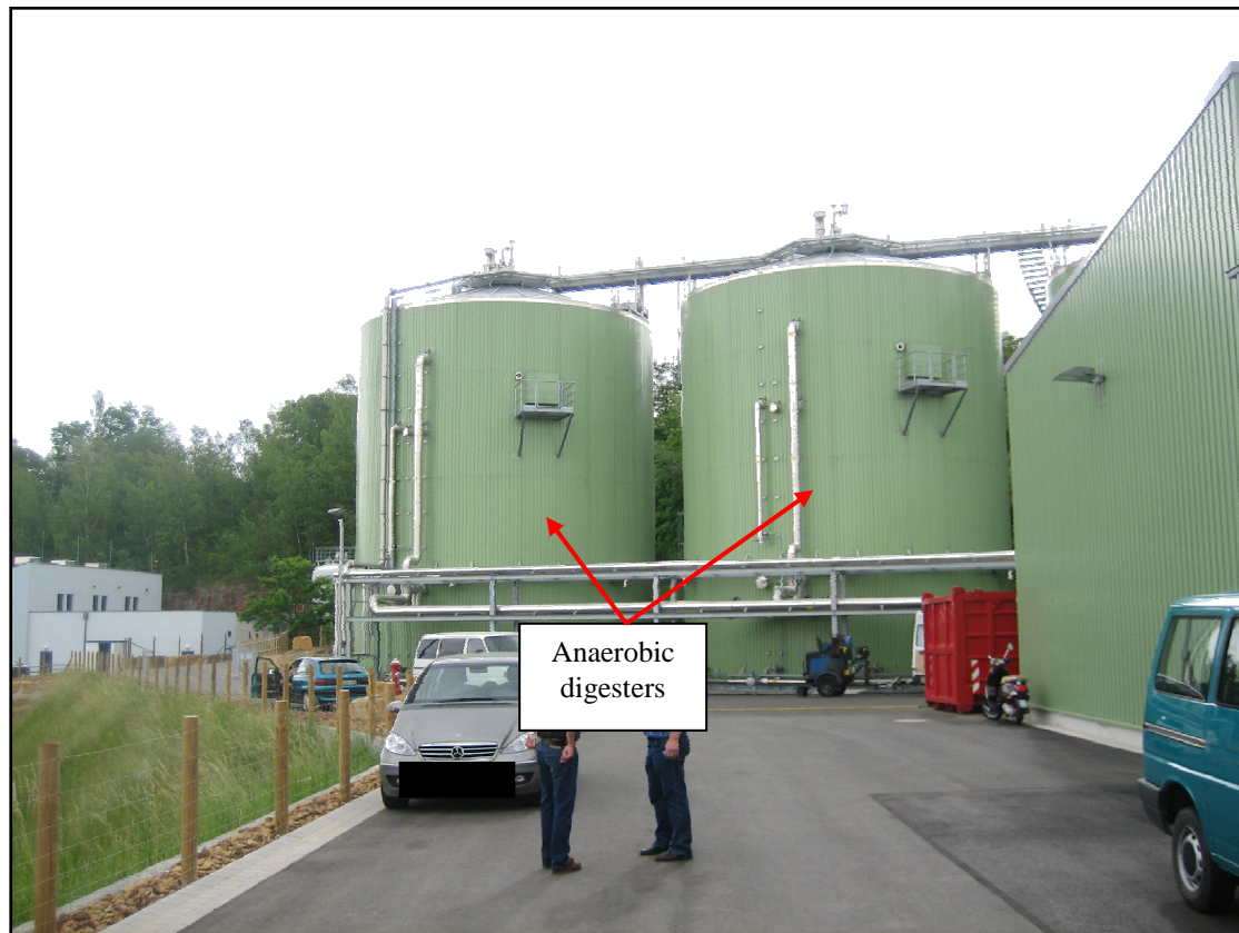
Figure 7 Two (of the three) anaerobic digesters
