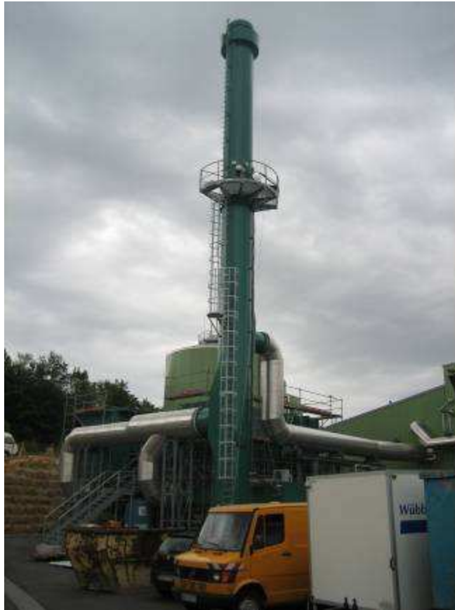
Figure 13 Thermal oxidation unit for exhaust gas treatment
