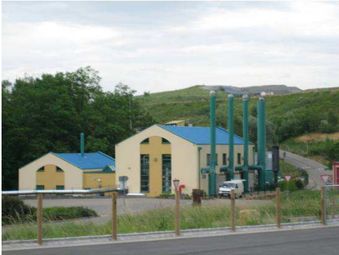
Figure 11 Biogas utilisation building
