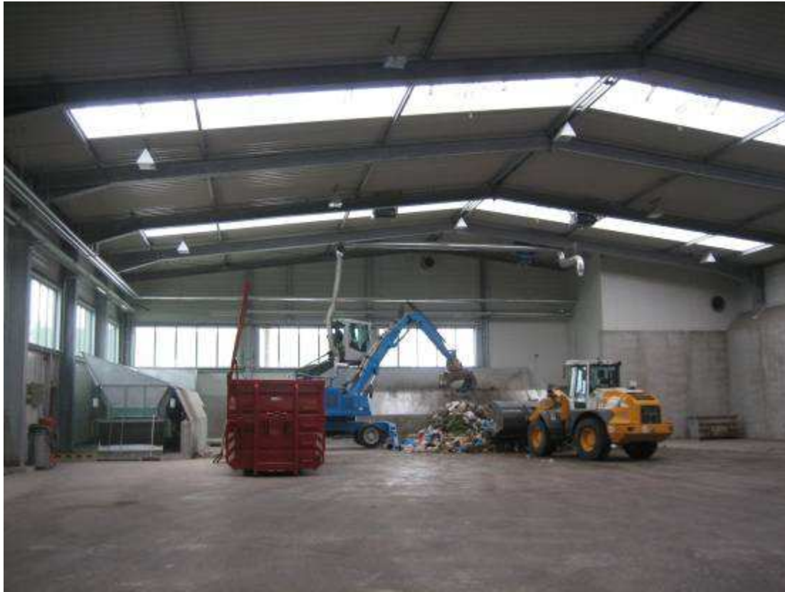
Figure 3 Waste reception hall
