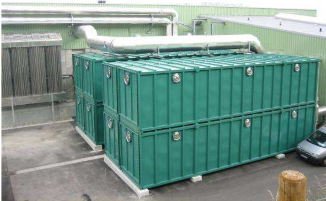
Figure 12 Biofilter for exhaust gas treatment
