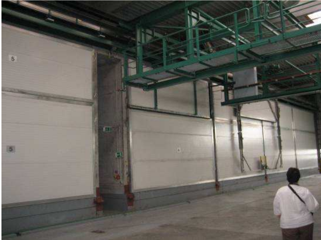
Figure 8 Biodrying bays (5 of 9)
