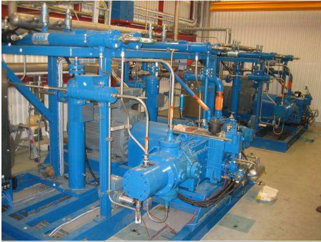
Figure 32 Compressors at Västerås Bus Depot
