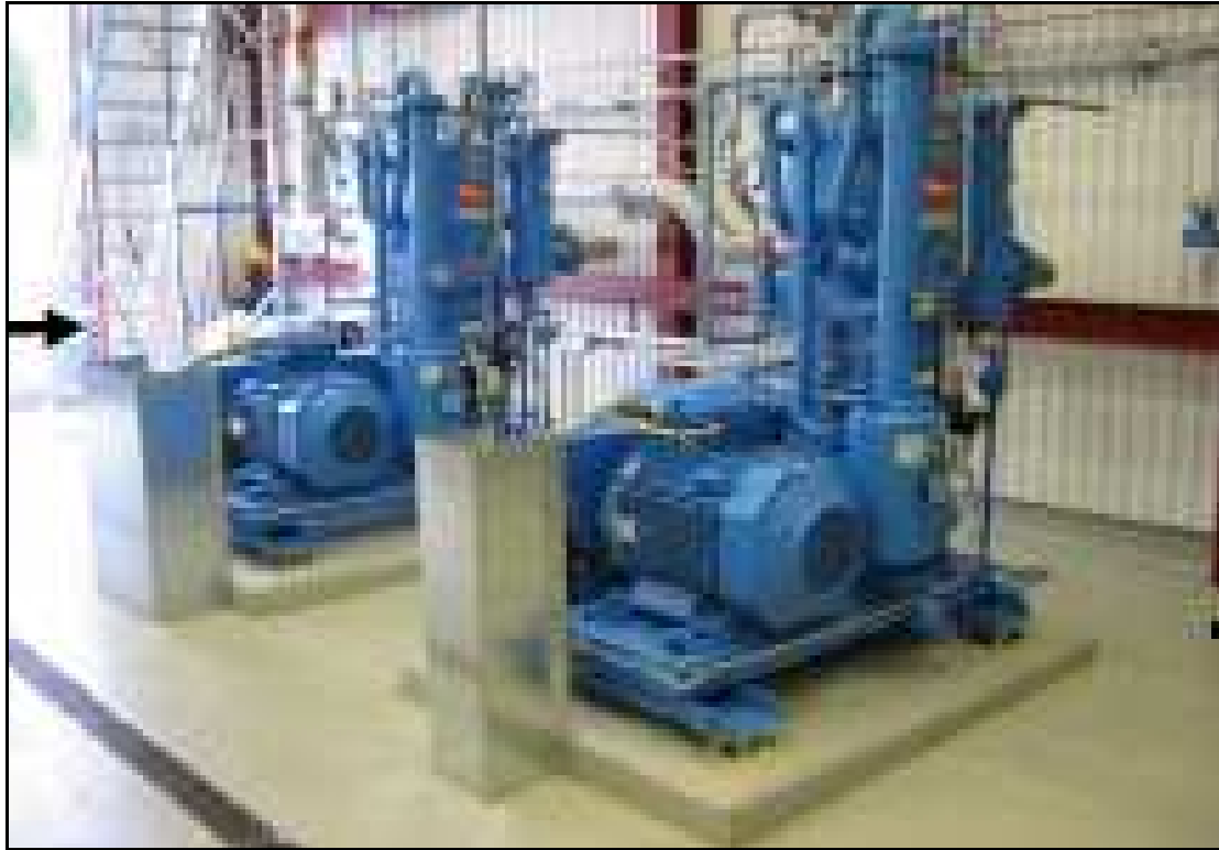
Figure 28 Compressor units (Ahrens, 2006)
