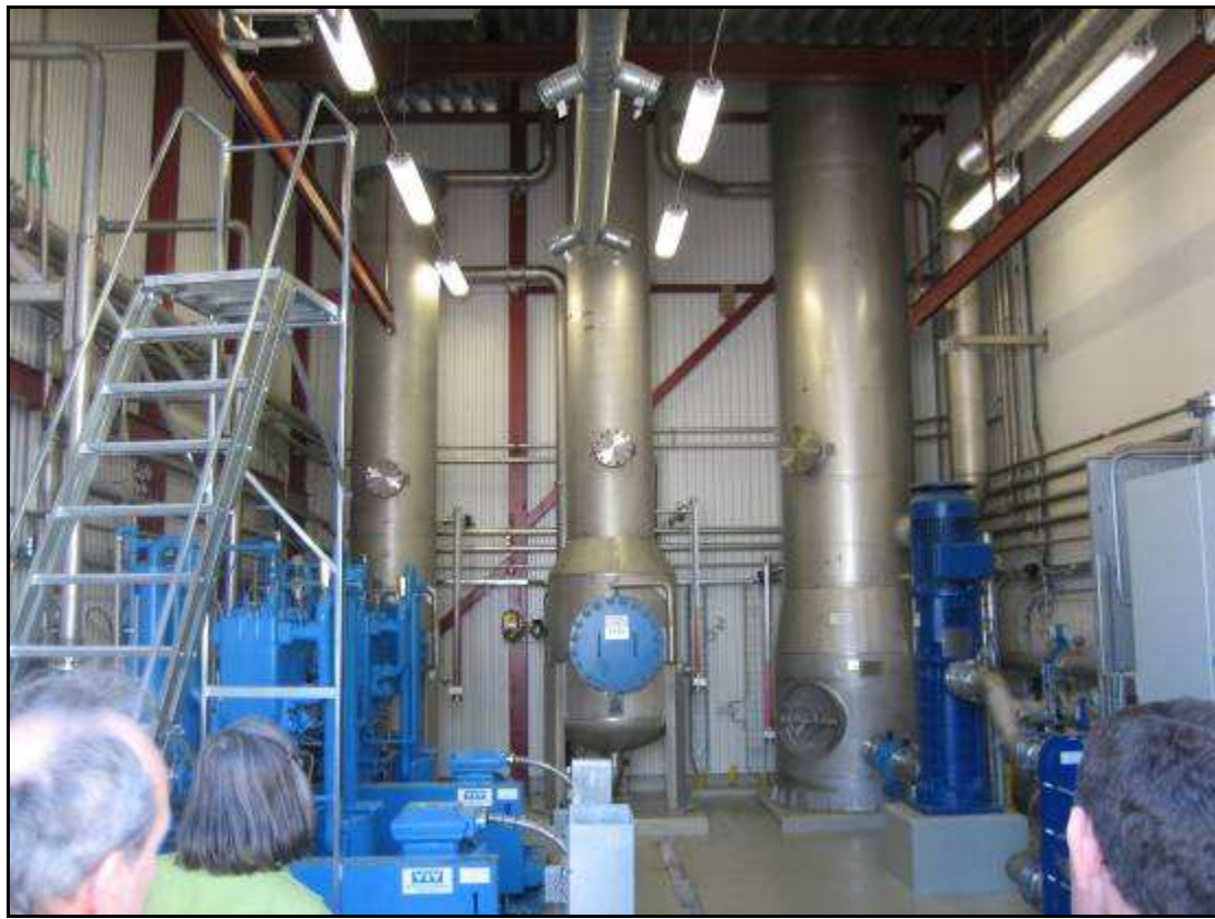
Figure 30 Inside of biogas upgrading building
