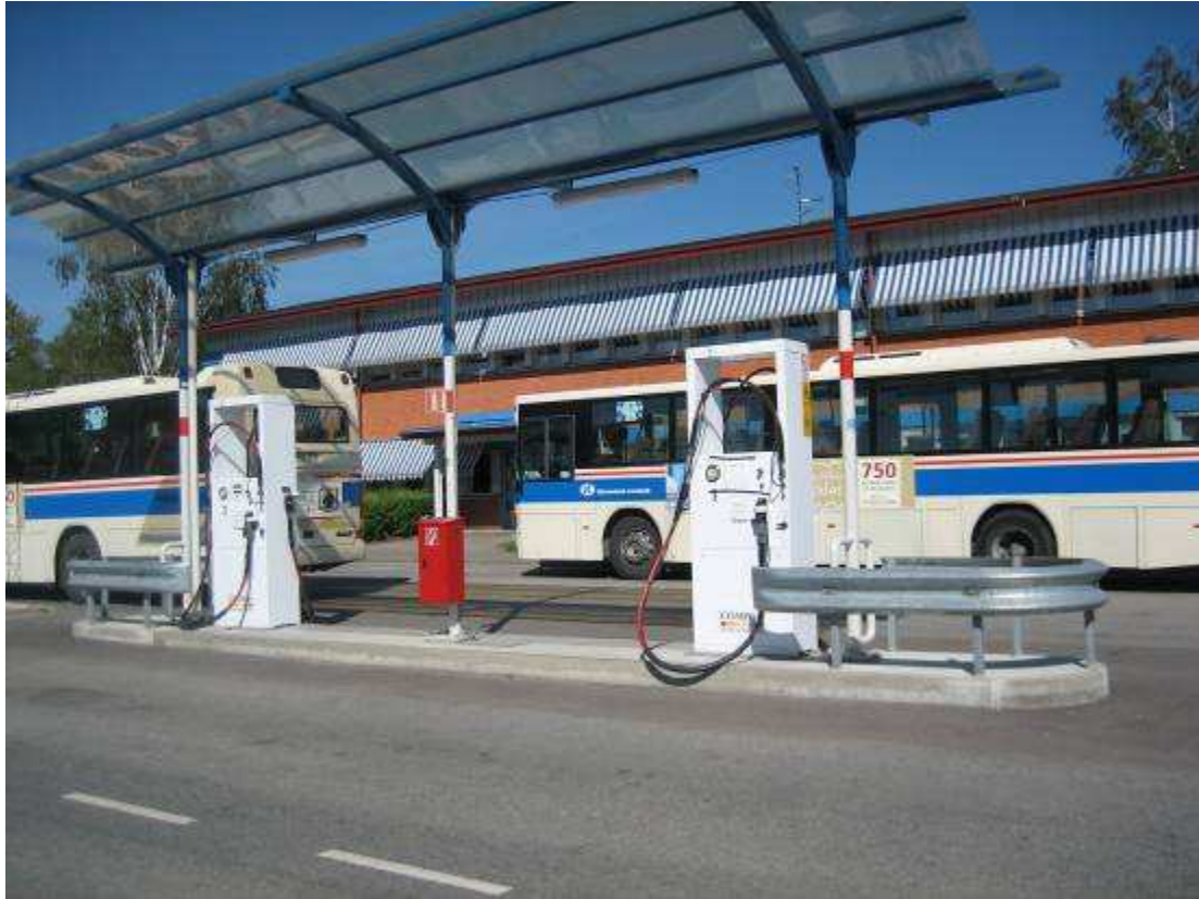
Figure 34 Biogas fuel pumps
