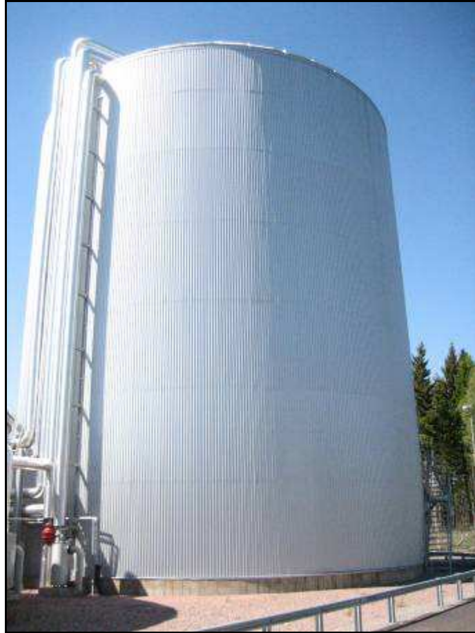
Figure 18 Anaerobic digester at Växtkraft plant
