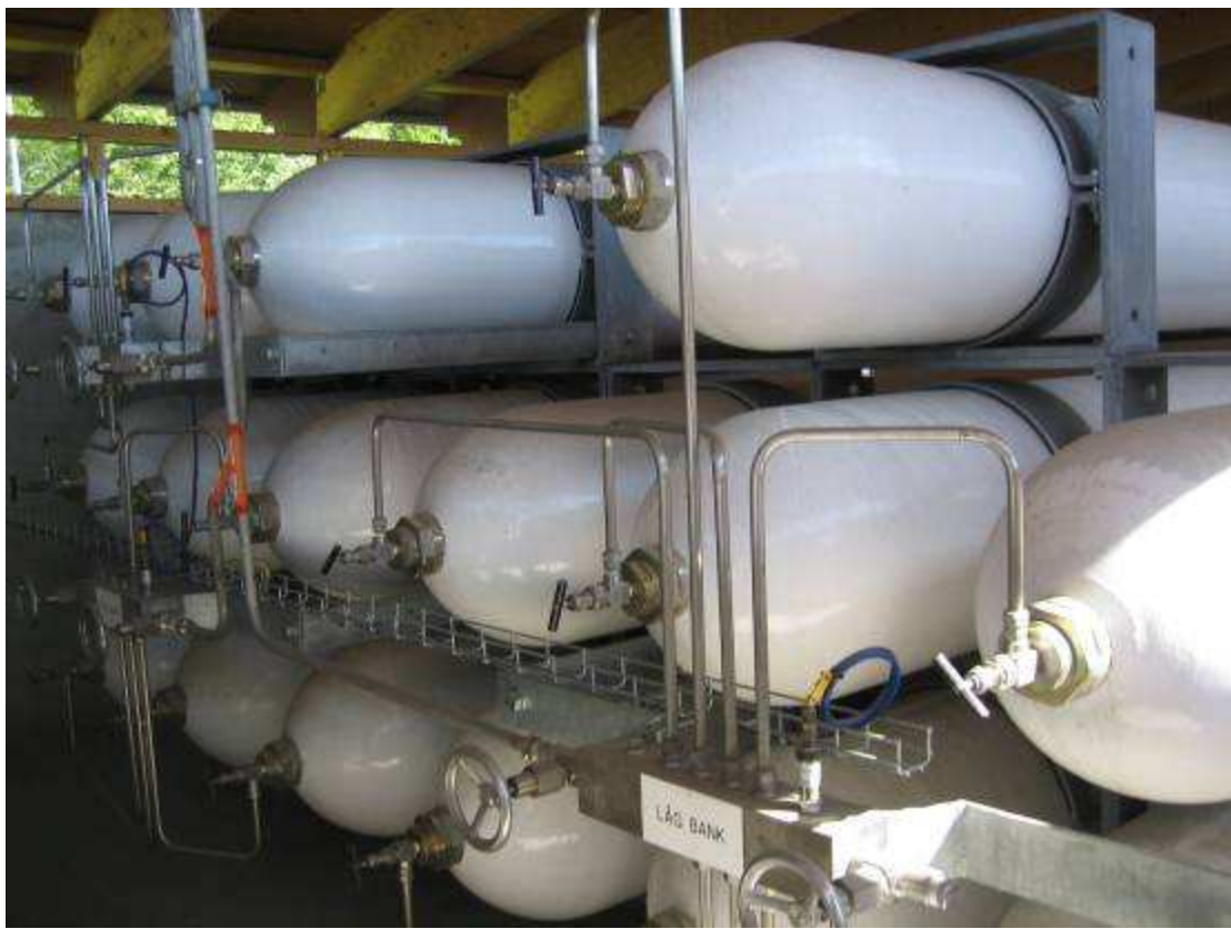
Figure 33 Biogas storage at Västerås Bus Depot
