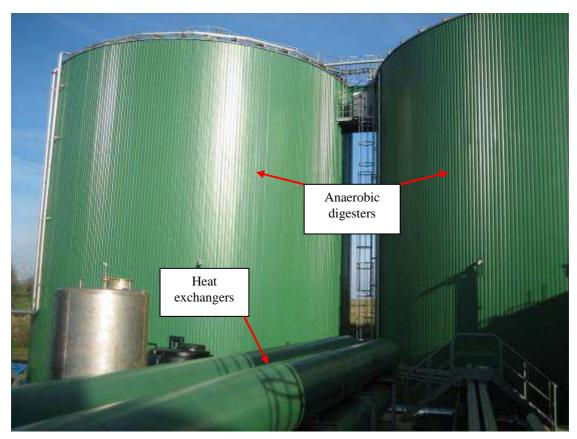
Figure 4Anaerobic digesters and heat exchangers
