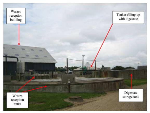
Figure 6Digestate storage tanks
