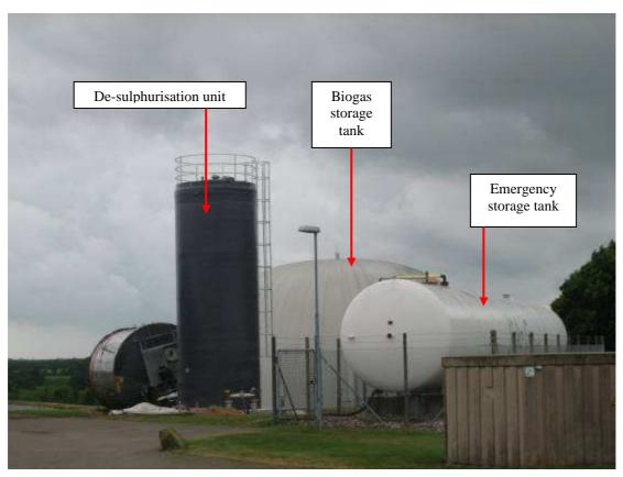
Figure 7 Biogas buffer/storage tank, emergency storage tank and desulphurisation unit
