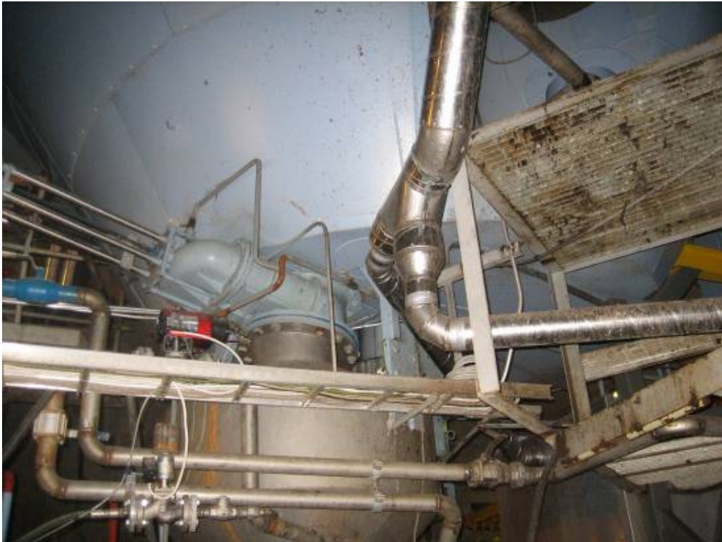
Figure 145 Bottom of the mix-separator
