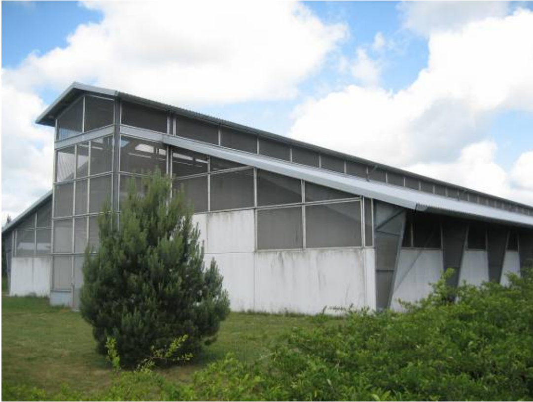
Figure 62 Digestate composting and storage hall
