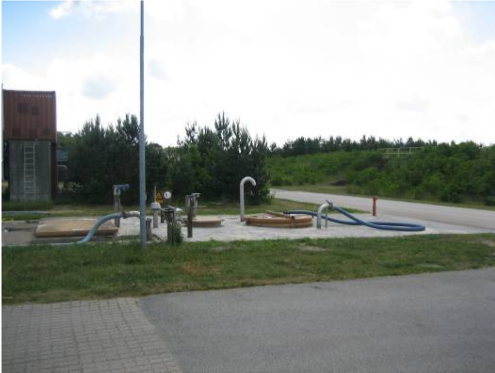
Figure 57 Industrial wastes reception tank
