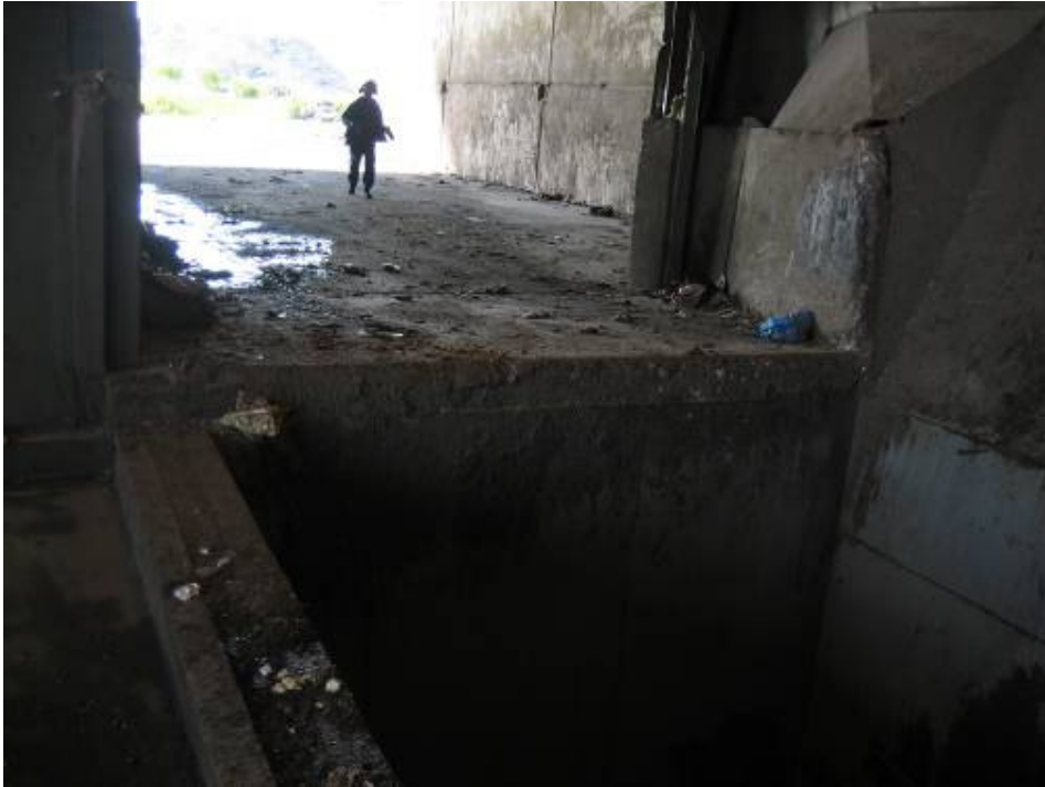
Figure 143 Emergency wastes reception area, dropping into wastes reception pit
