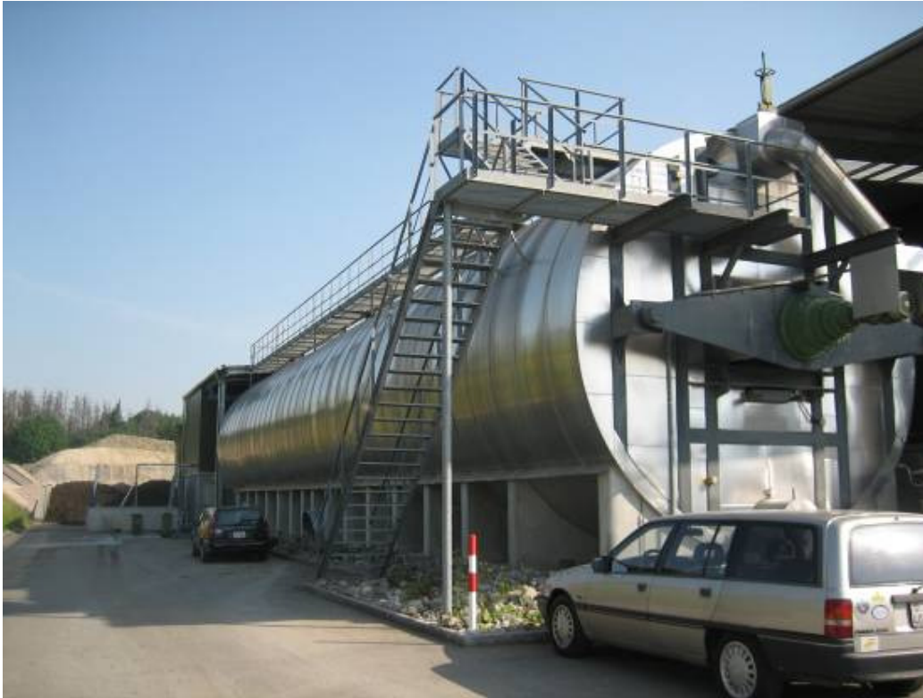
Figure 90 Kompogas anaerobic digester at Oetwil Am See
