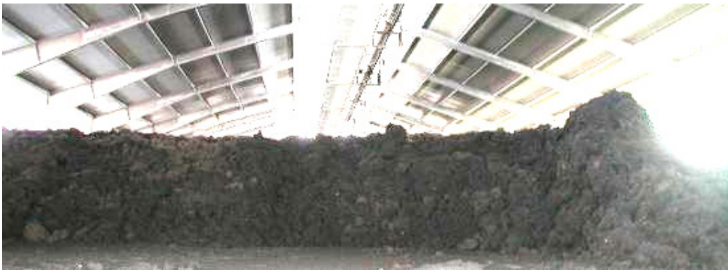
Figure 61 Inside digestate storage building (Bro, 2006)
