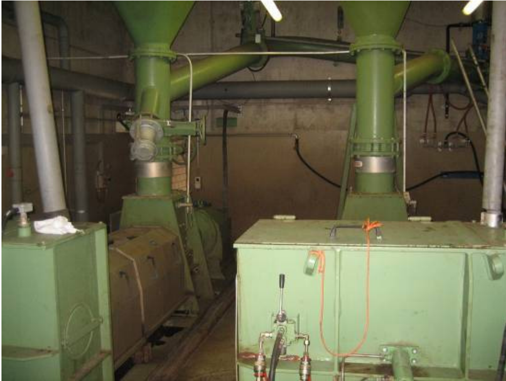
Figure 98 Screw presses
