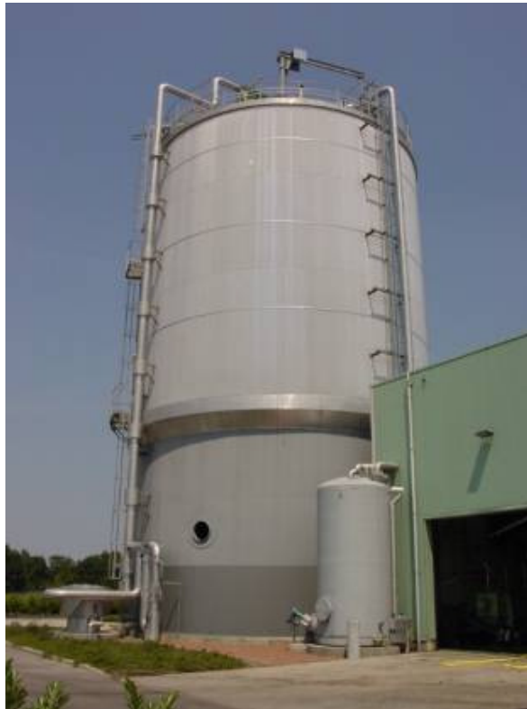
Figure 49 Dranco anaerobic digester at Brecht
