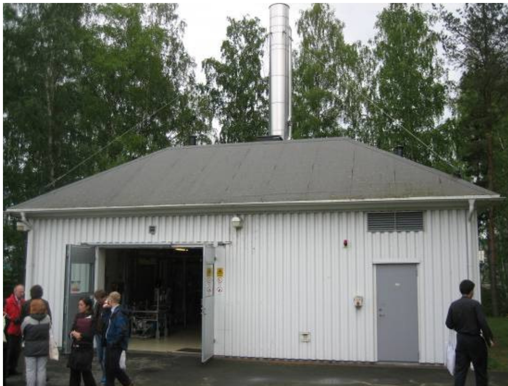
Figure 73 Biogas upgrading unit at Simsholmen
