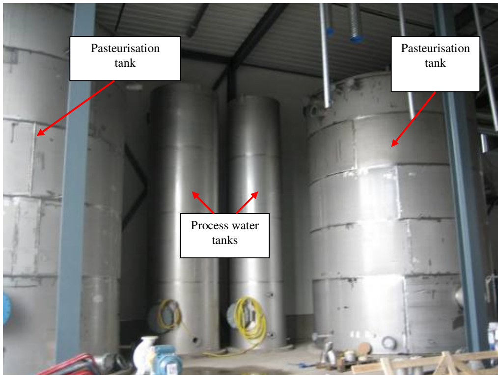
Figure 69 Pasteurisation tanks and process water tanks at Torsvik
