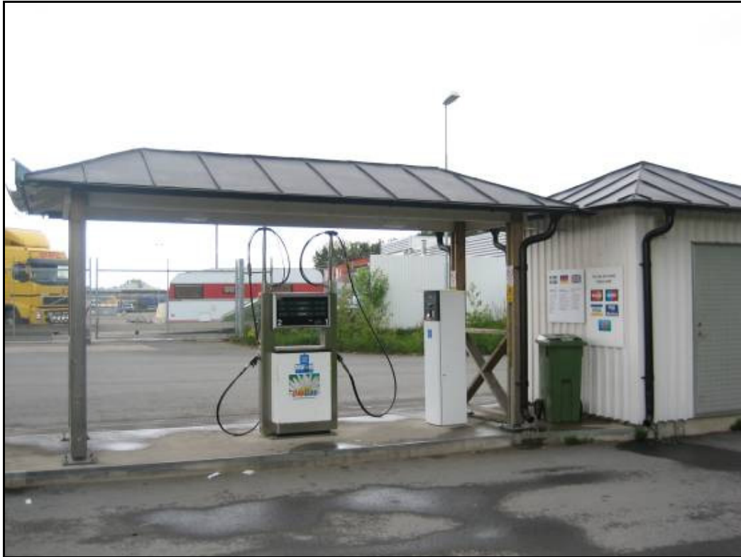
Figure 16 Public biogas filling station at Simsholmen (Jonkoping, Sweden)
