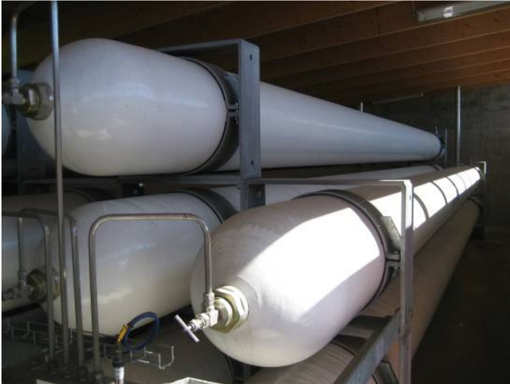
Figure 13 Compressed biogas storage tanks
