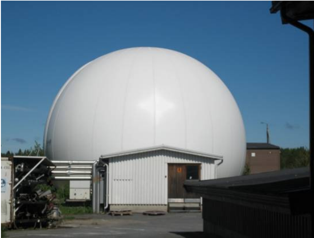
Figure 147 Biogas storage tank
