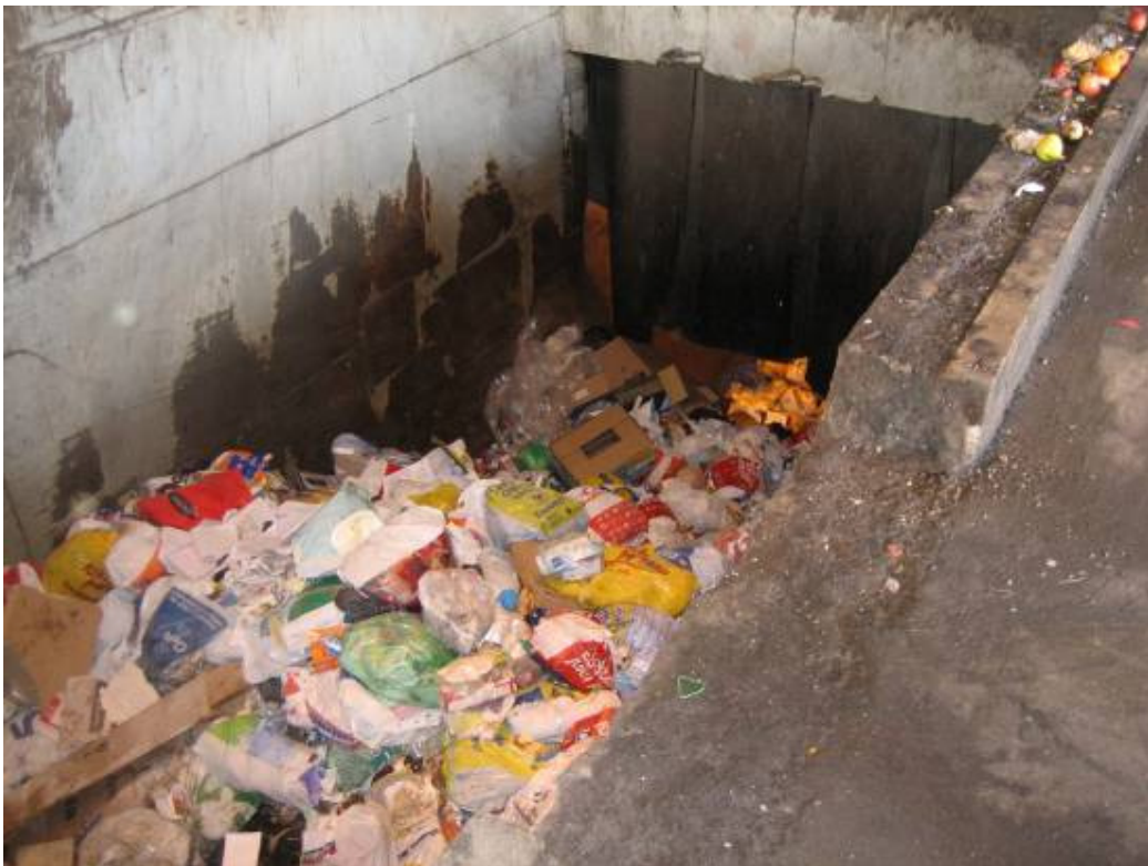
Figure 142 Wastes reception pit at Stormossen
