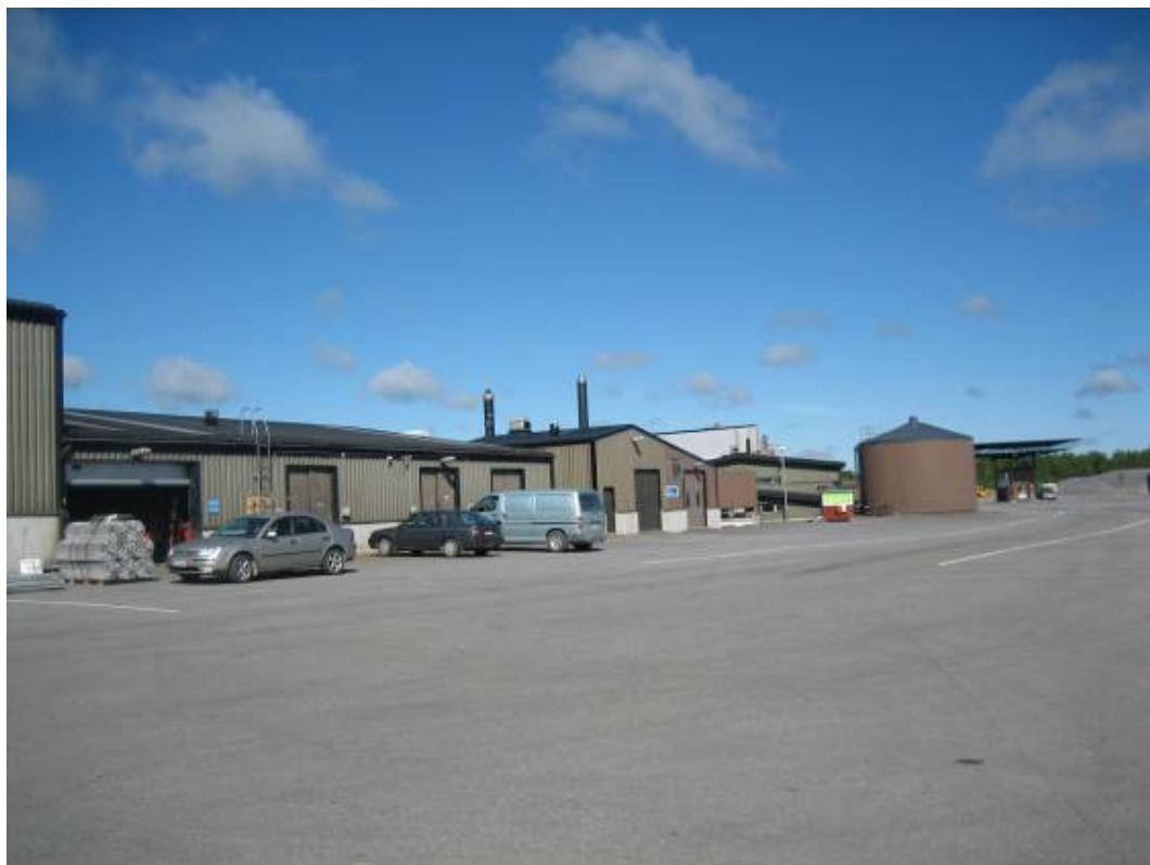
Figure 139 Stormossen wastes treatment plant
