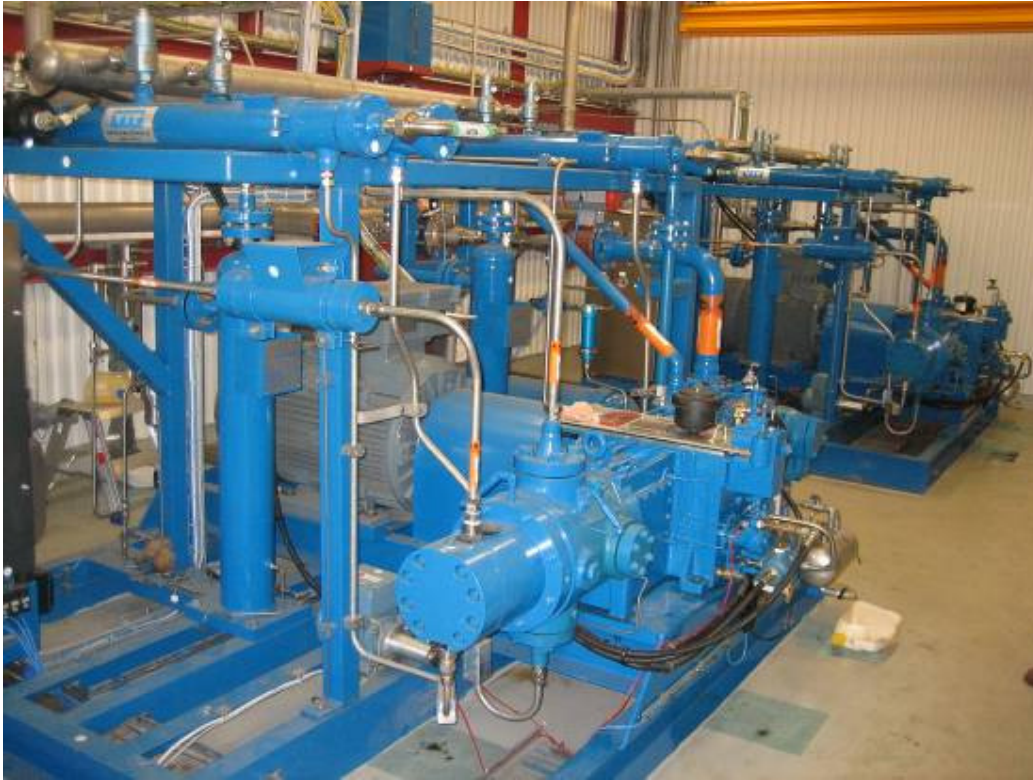
Figure 12 Compressors at Västerås Bus Depot
