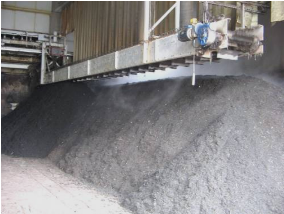
Figure 51 Inside in-vessel composting hall
