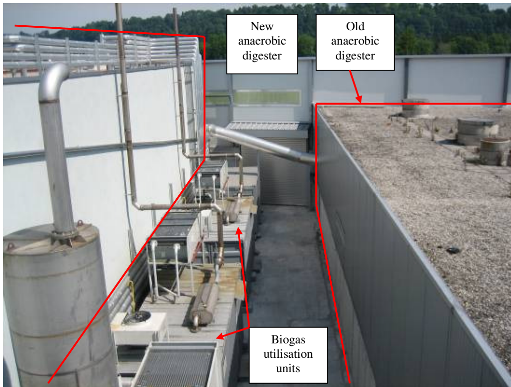
Figure 97 Two anaerobic digesters at Niederuzwil
