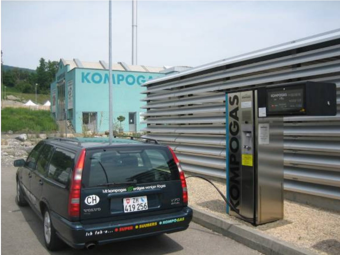
Figure 113 Biogas filling station at Otelfingen
