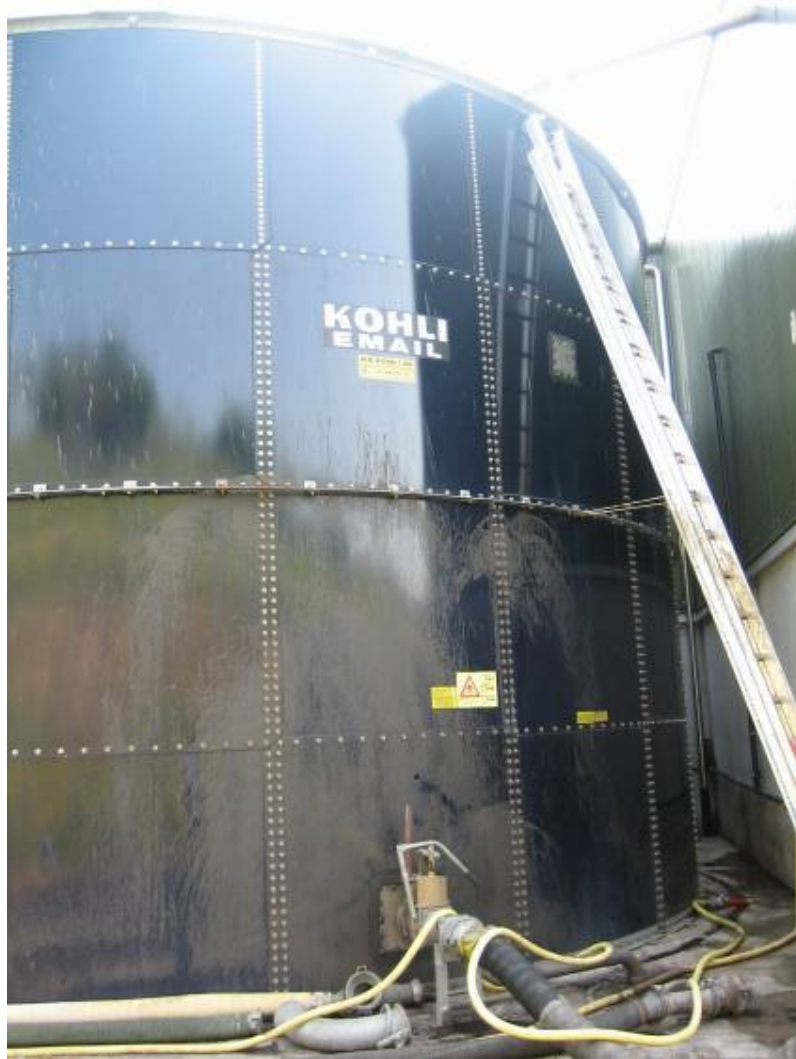
Figure 91 Liquid fertiliser storage tank
