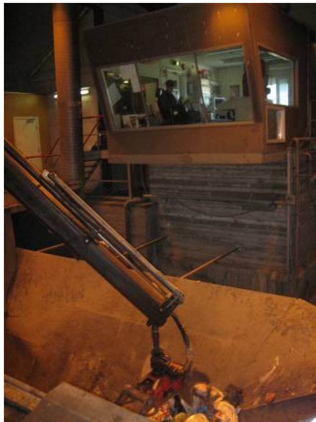
Figure 144 Mini-crane for removal of large non-organic contaminants
