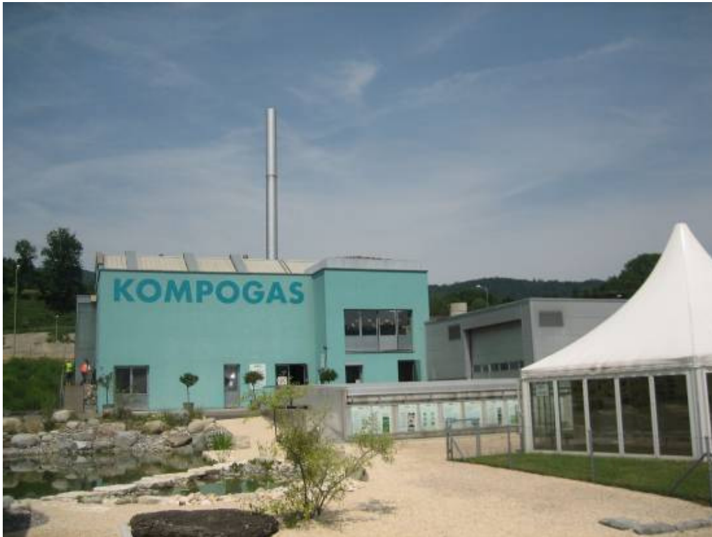
Figure 104 Kompostogas biowastes treatment plant at Otelfingen
