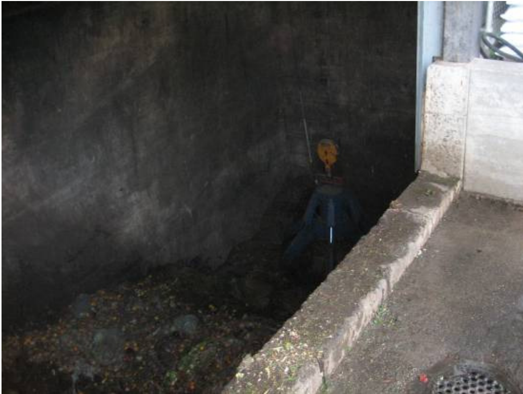
Figure 95 Wastes reception pit
