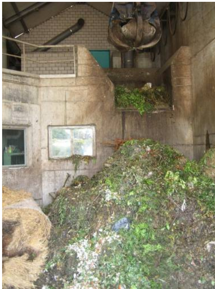
Figure 108 Wastes reception pit and picking crane
