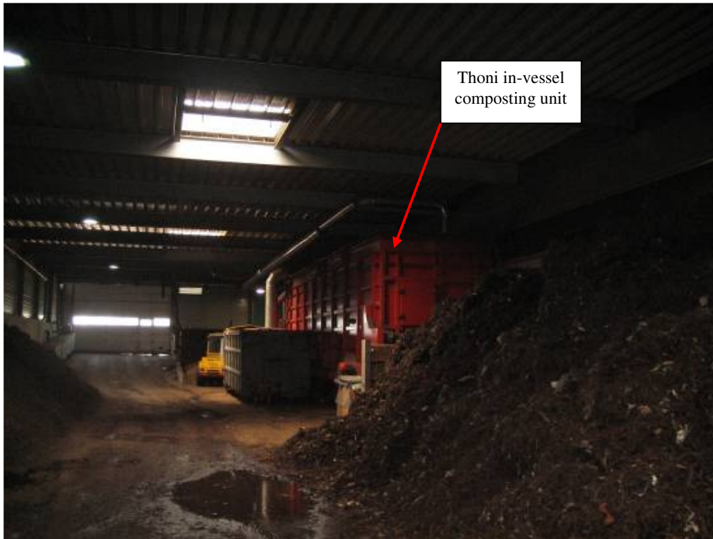
Figure 109 Thoni in-vessel composting system at Otelfingen
