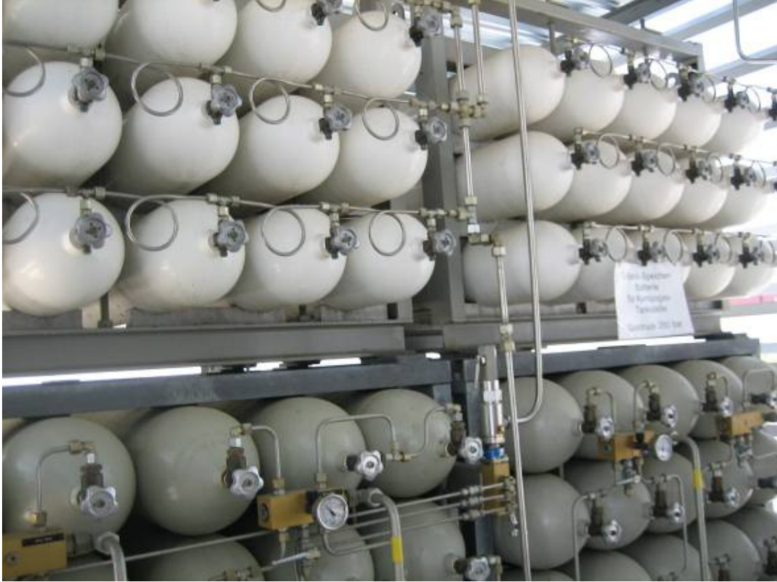
Figure 112 Biogas storage at filling station at Otelfingen
