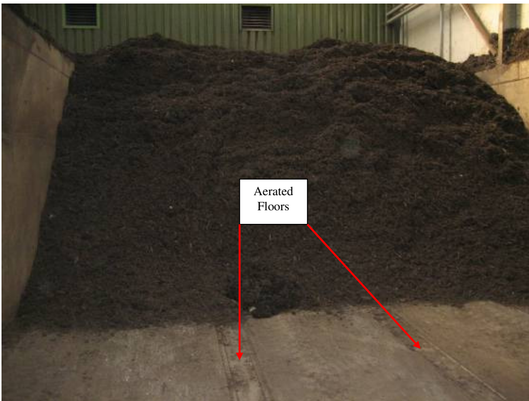
Figure 93 Aerated floors in covered composting bays
