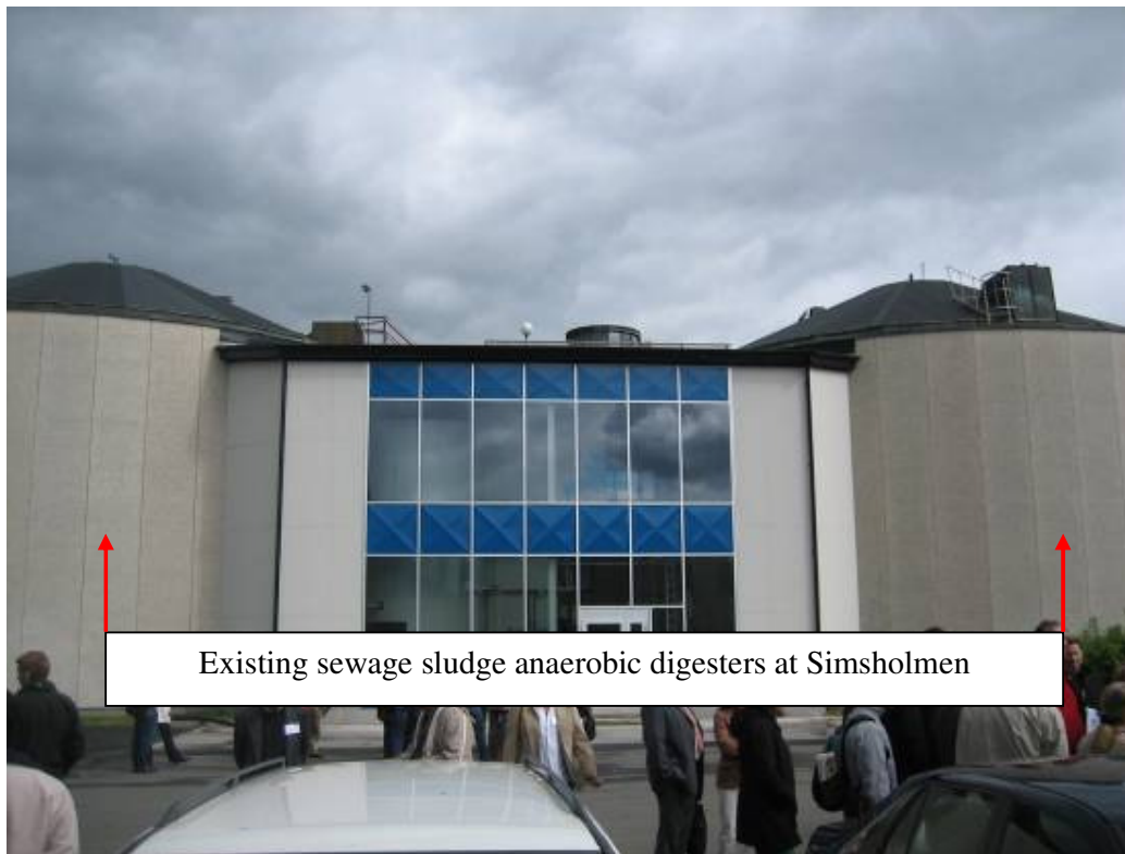
Figure 71 Anaerobic digesters at Simsholmen
