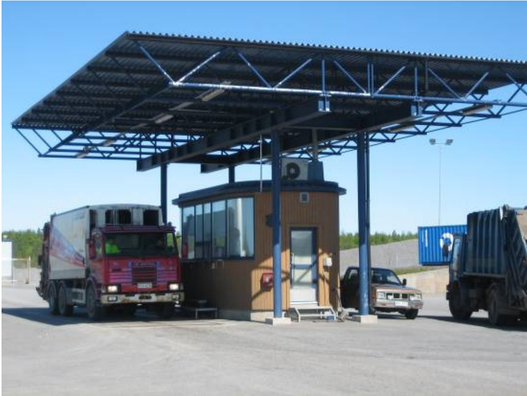
Figure 141 Weighbridge at Stormossen
