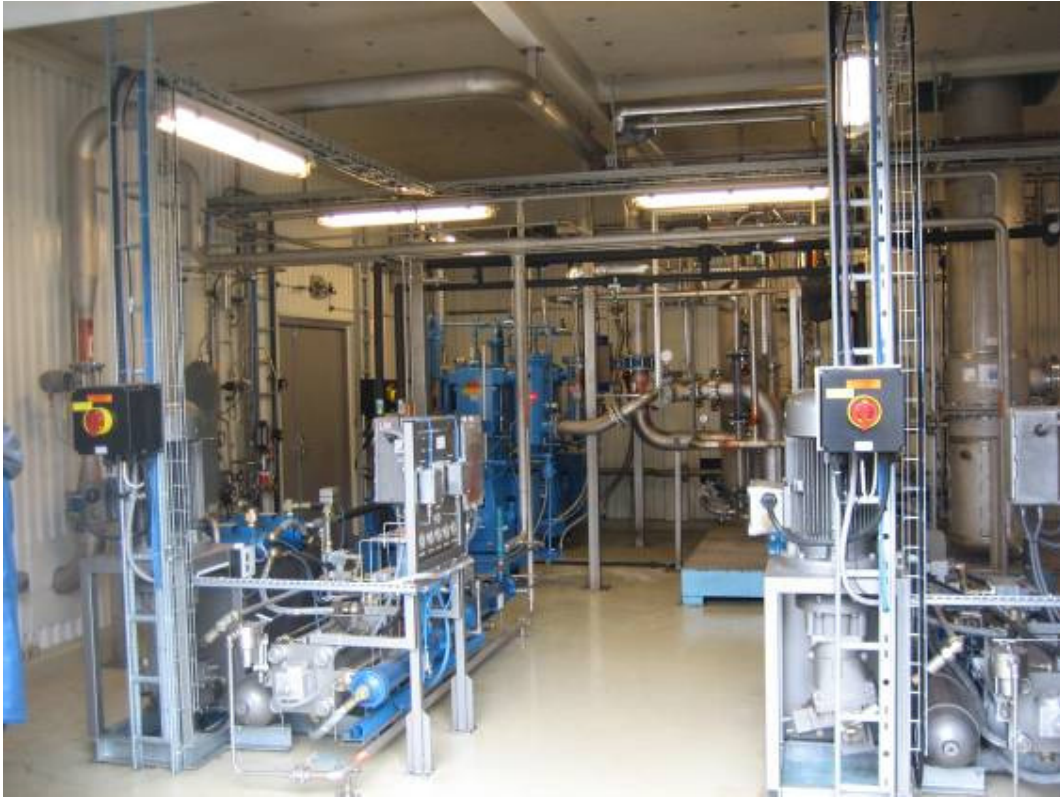
Figure 74 Inside biogas upgrading unit
