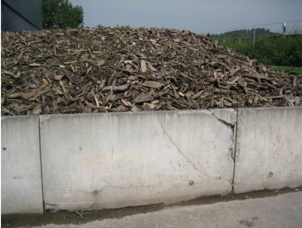
Figure 103 Biofilter at Niederuzwil
