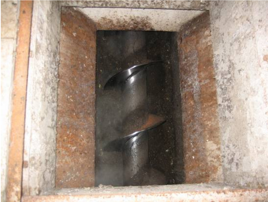
Figure 130 Screw pump to conveyor belt to in-vessel composter
