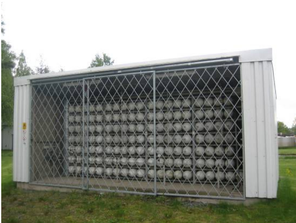
Figure 75 Upgraded biogas storage at Simsholmen
