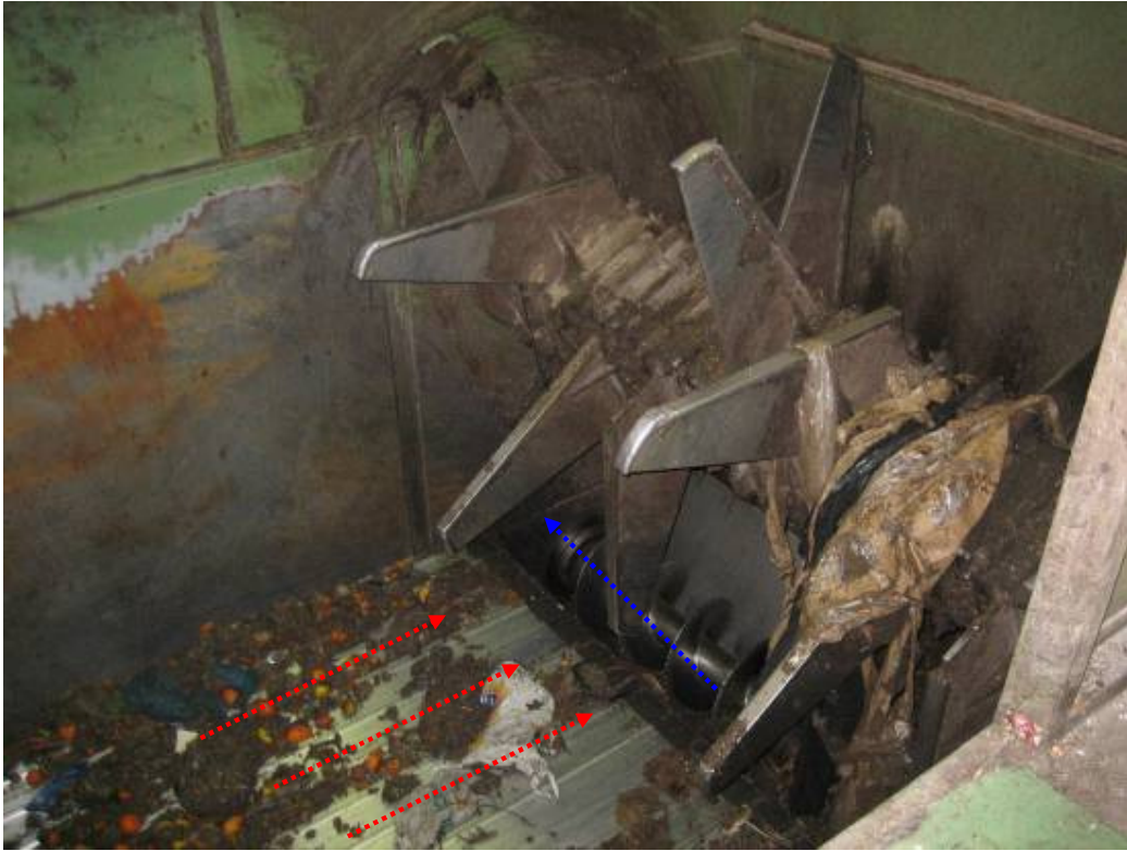
Figure 122 Wastes reception pit
