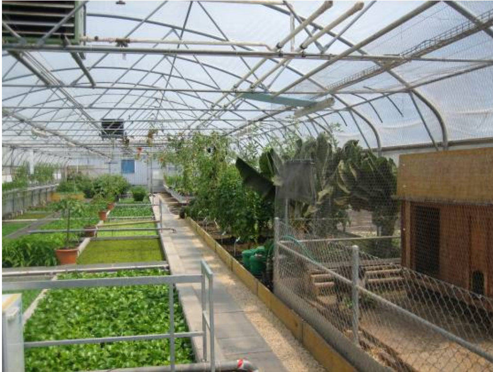
Figure 106 Inside greenhouse at Otelfingen
