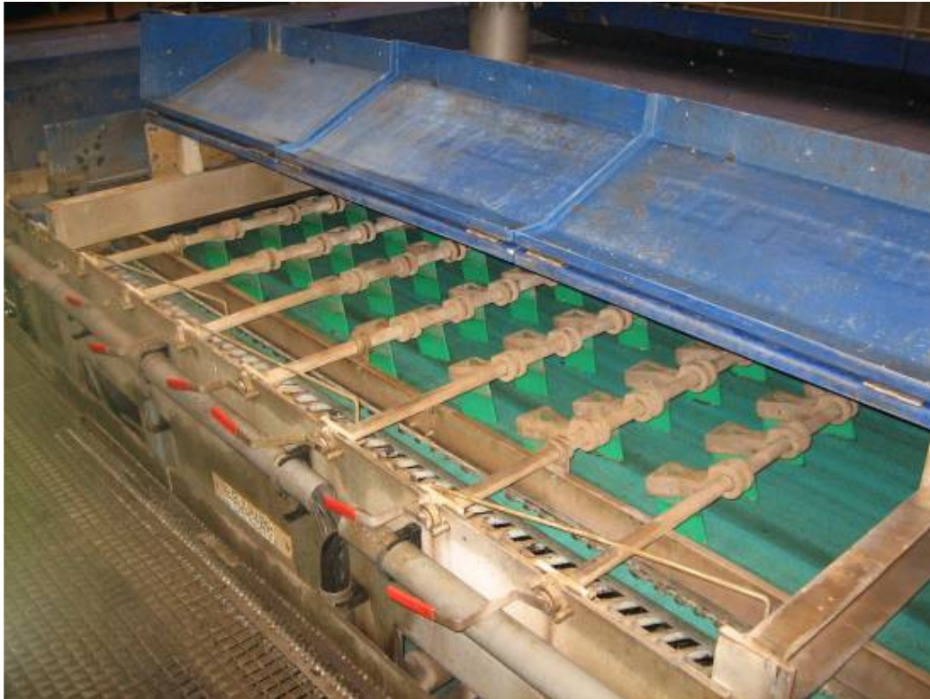
Figure 214 Belt-presses for de-watering digestate
