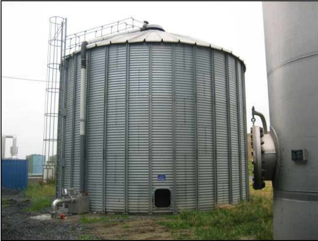
Figure 230 Biogas buffer/storage tank
