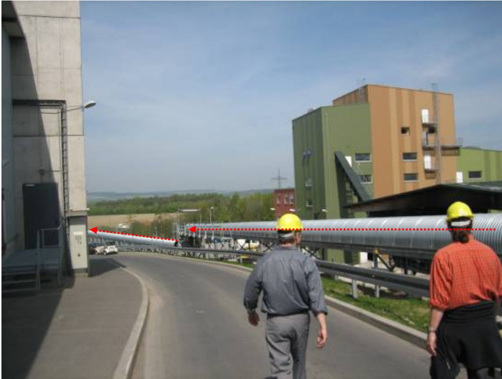
Figure 194 Conveyor belt from IVC to landfill site
