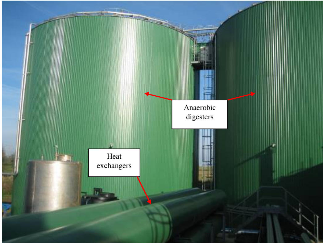
Figure 265 Anaerobic digesters and heat exchangers
