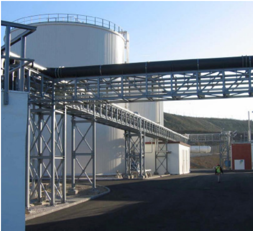
Figure 288 Anaerobic digesters at the ETVO site (Linde Promotional Information)
