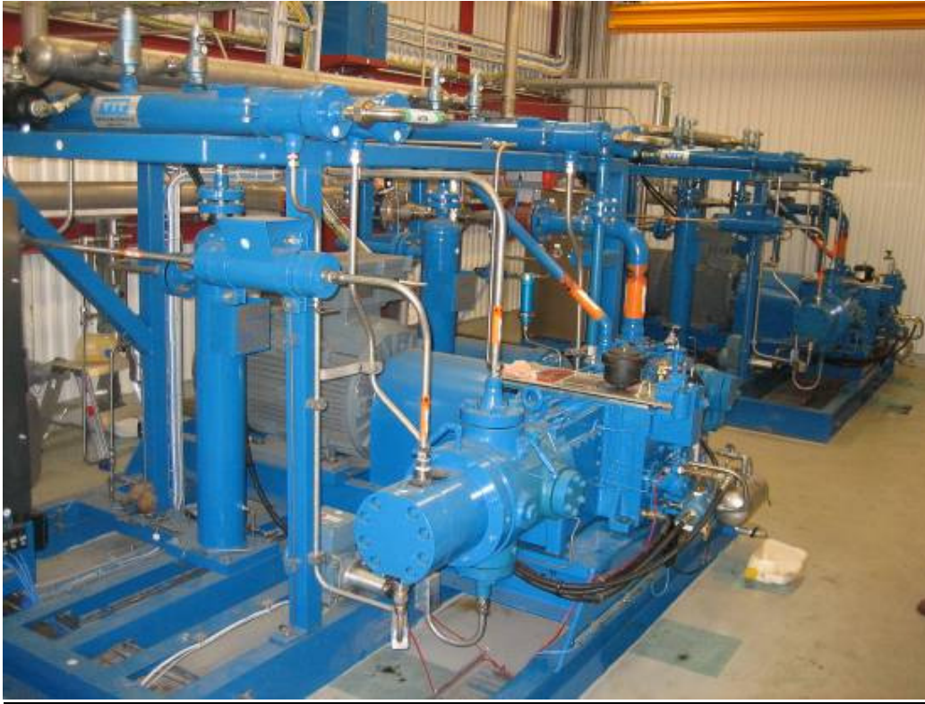
Figure 182 Compressors at Västerås Bus Depot
