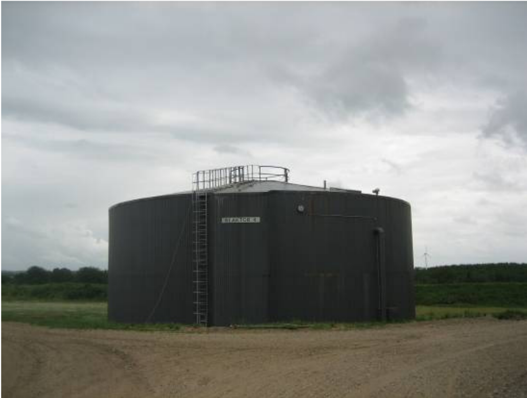
Figure 279 Anaerobic digester at Lintrup
