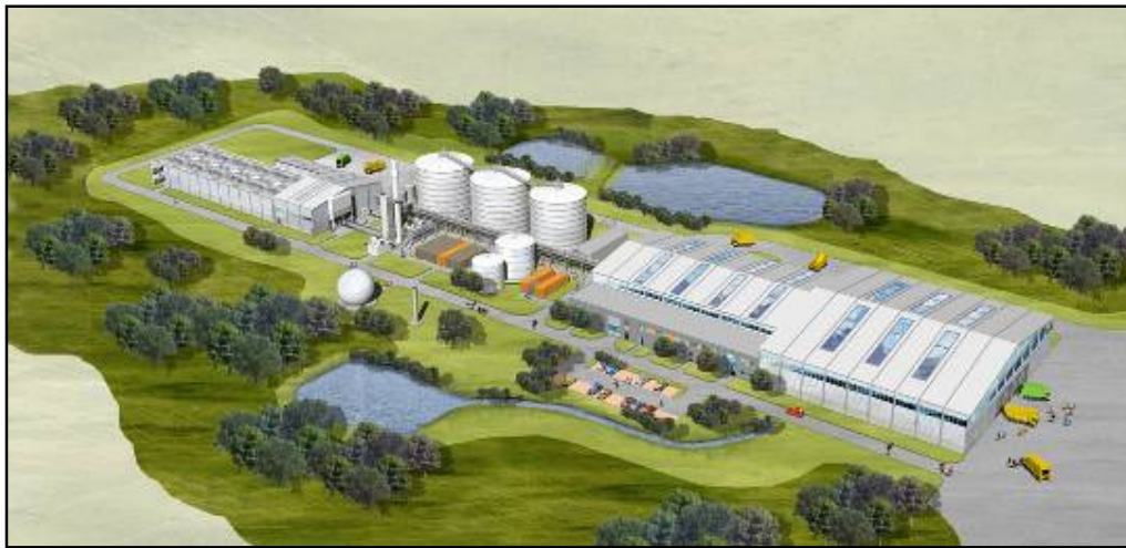
Figure 297 Aerial photograph of Luebeck MBT Plant (Haase website, accessed July 2006)
