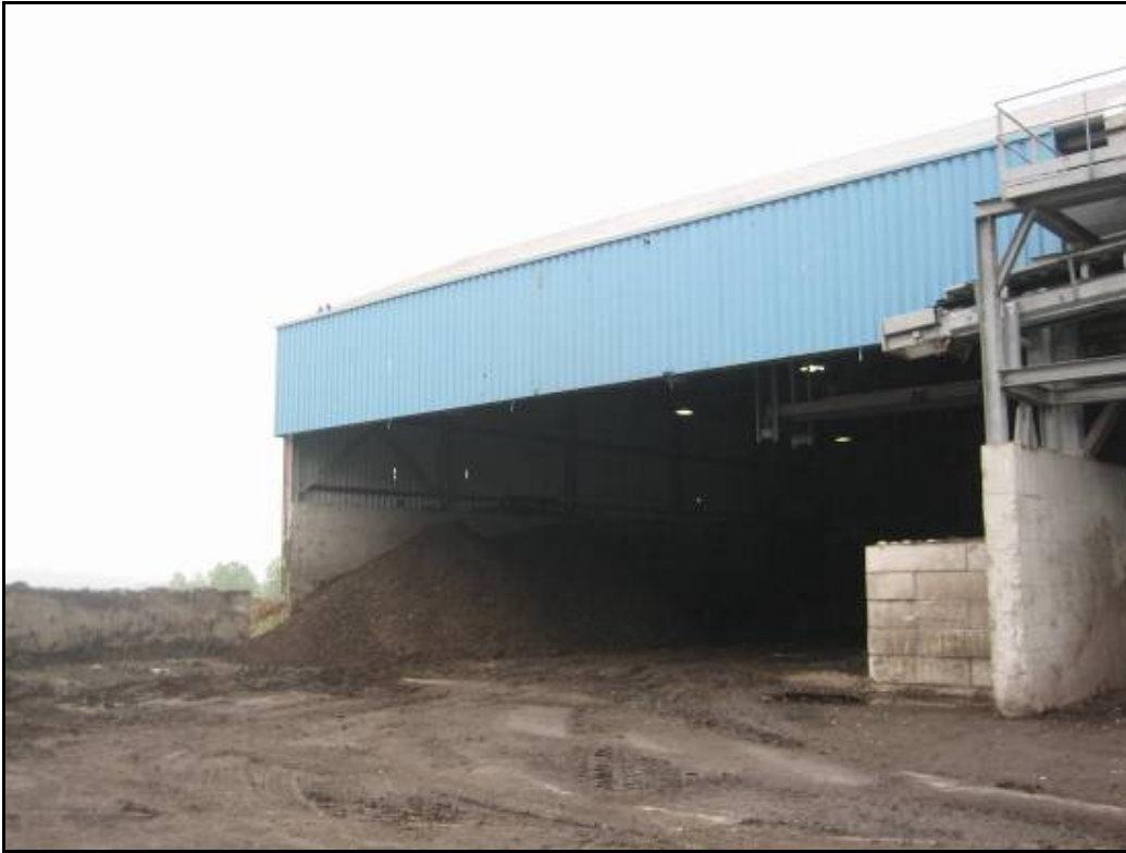
Figure 228 Compost storage hall
