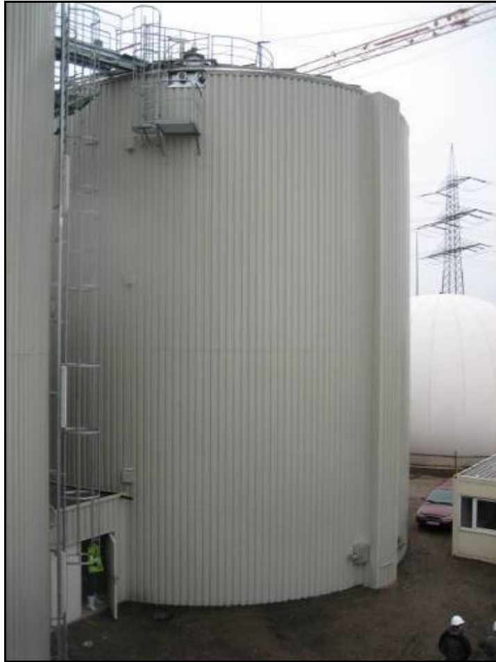
Figure 246 Anaerobic digester at Saschenhagen (one of four)
