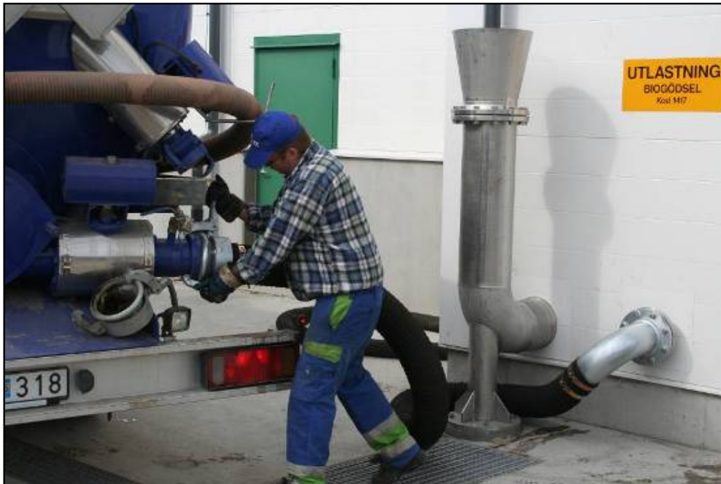
Figure 170 Liquid digestate transport from site (Pettersson, 2006)
