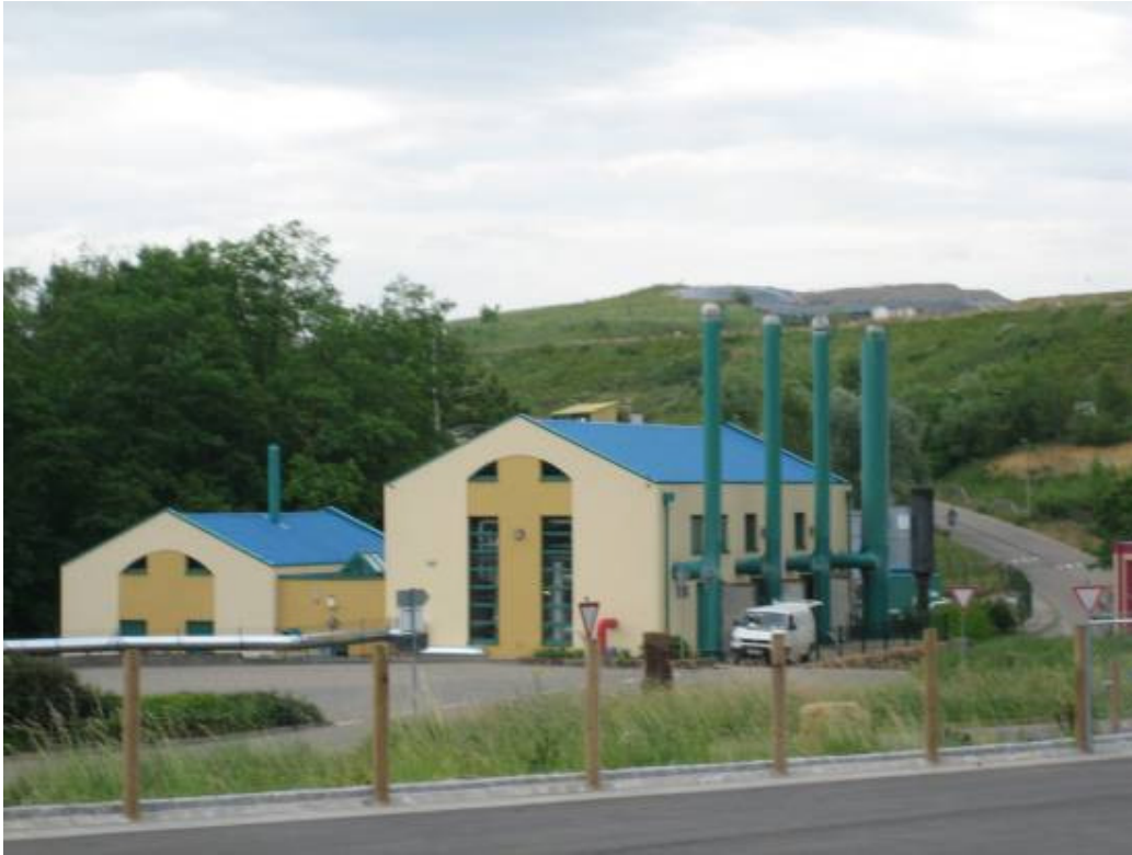
Figure 258 Biogas utilisation building
