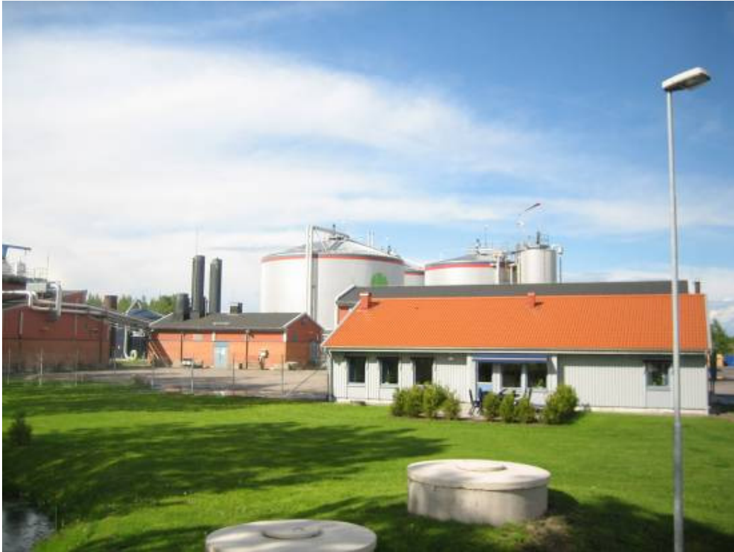
Figure 274 Linköping Biogas Plant
