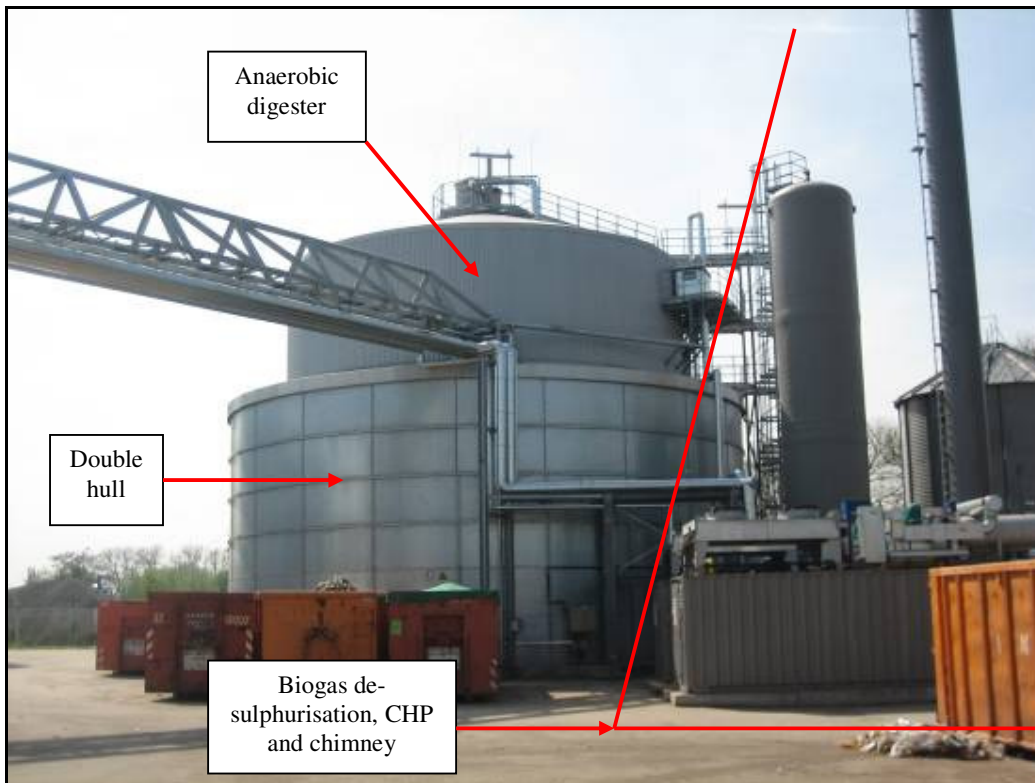
Figure 206 Anaerobic digester at Heilbronn
