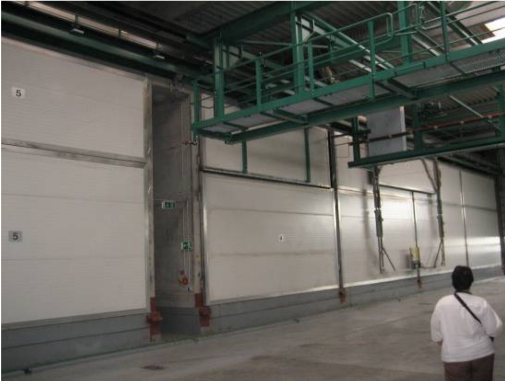
Figure 255 Biodrying bays (5 of 9)
