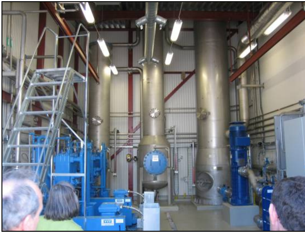
Figure 180 Inside of biogas upgrading building
