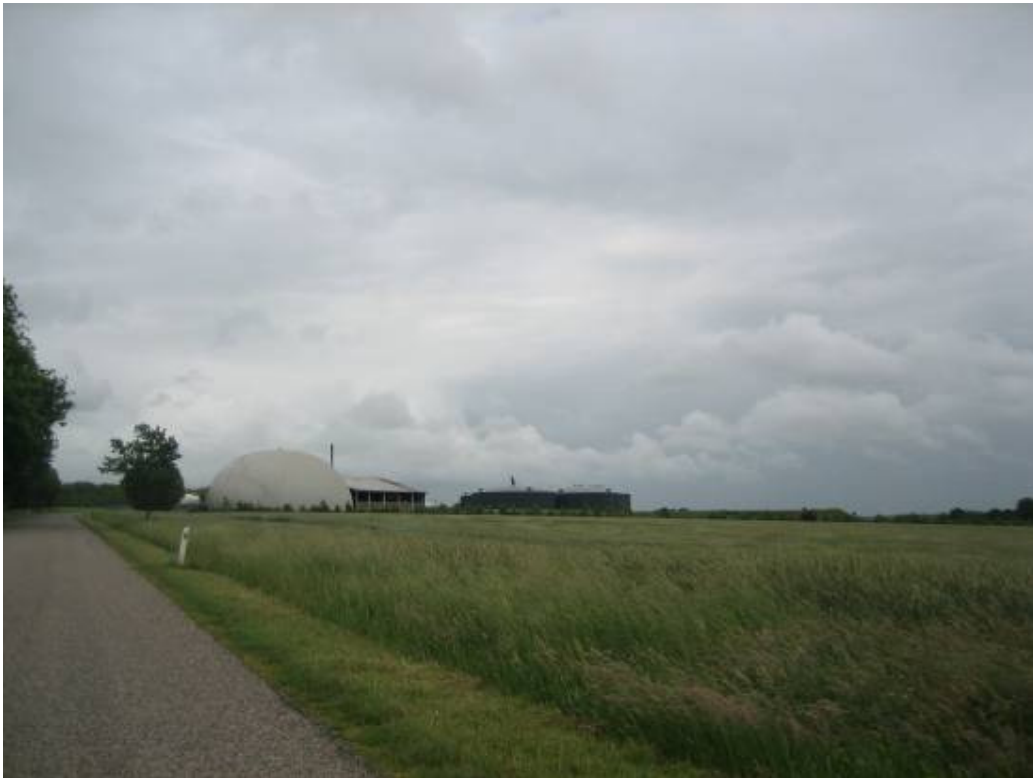
Figure 282 Lintrup Biogas Plant
