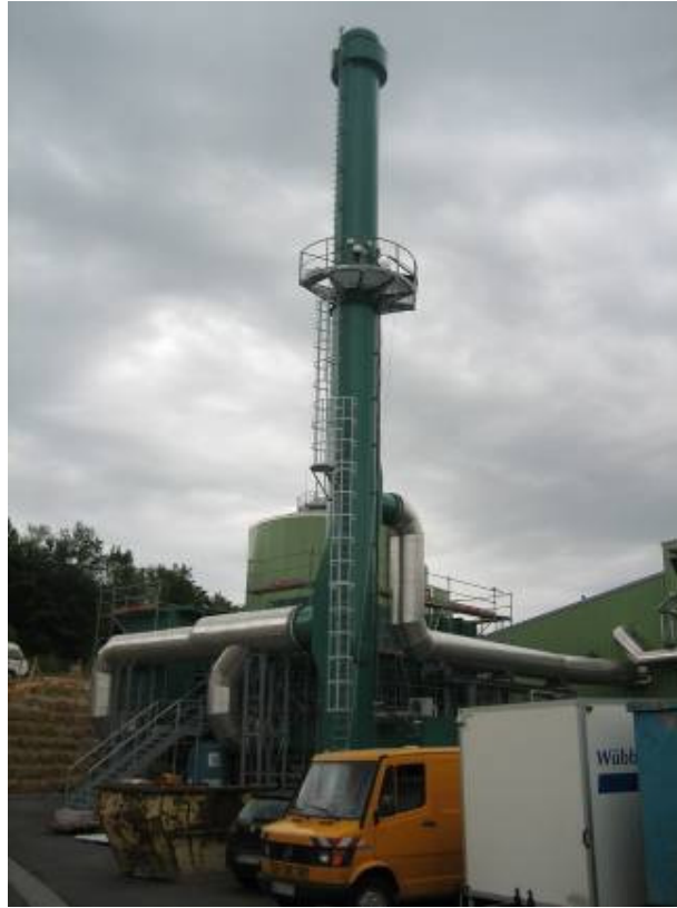
Figure 260 Thermal oxidation unit for exhaust gas treatment
