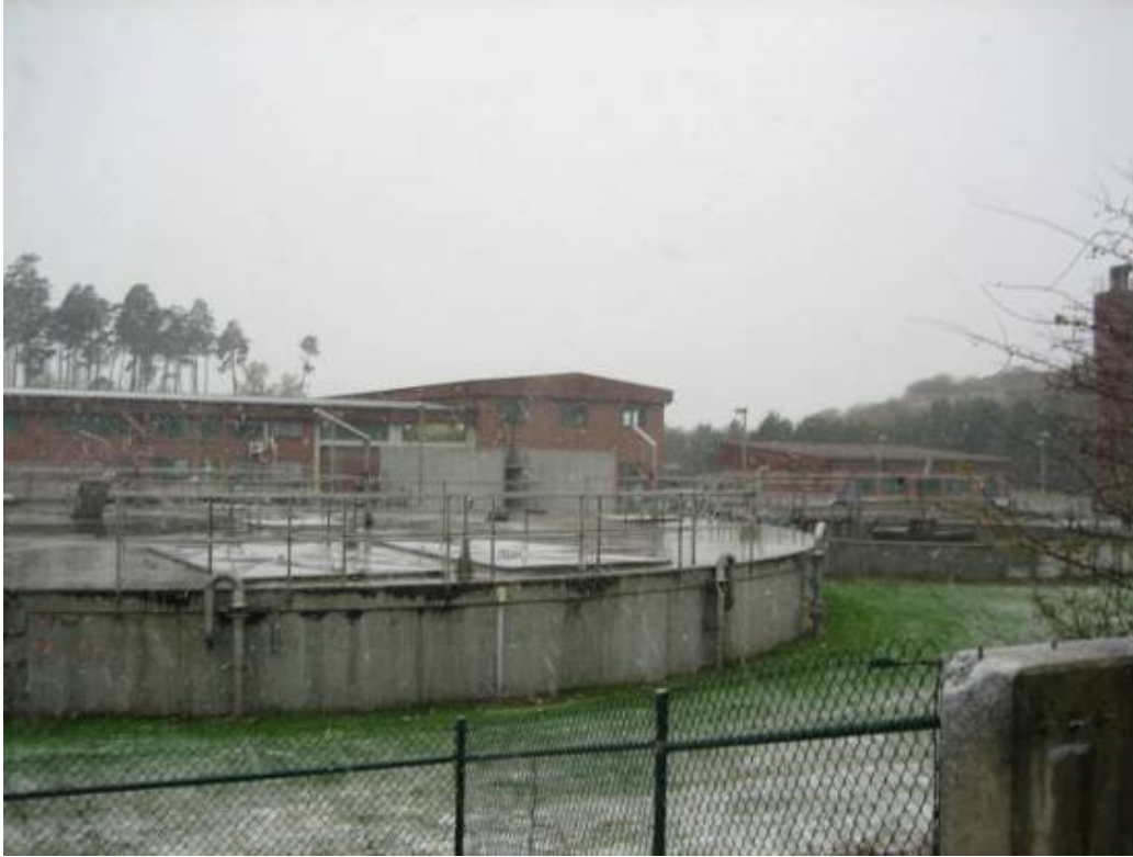
Figure 243 Wastewater treatment plant
