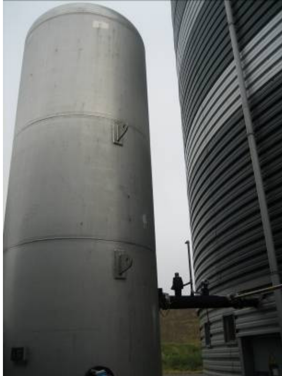
Figure 224 Biogas pressurisation unit
