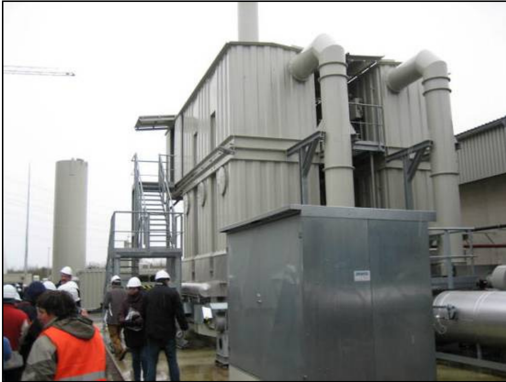
Figure 247 Exhaust gas thermal oxidation plant and chimney
