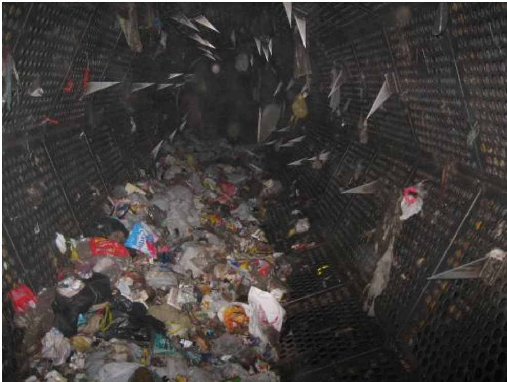
Figure 221 Inside trommel sieves
