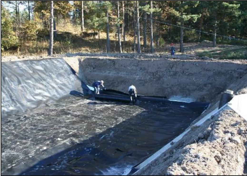
Figure 172 On-farm liquid digestate storage tank (Pettersson, 2006)
