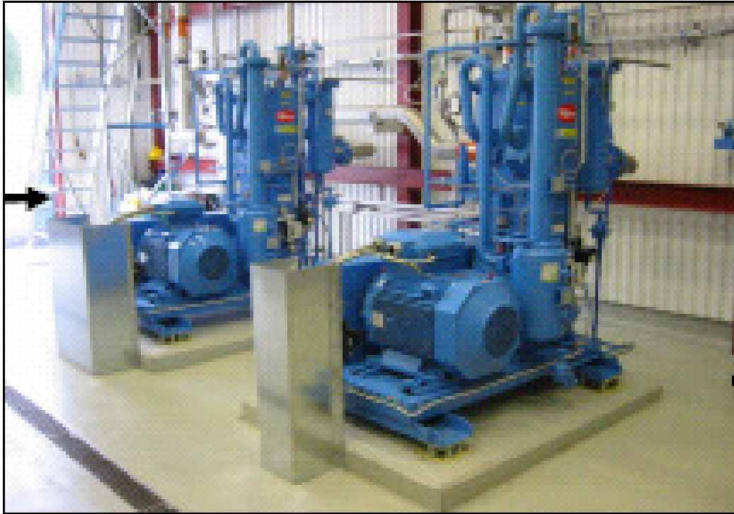
Figure 178 Compressor units (Ahrens, 2006)
