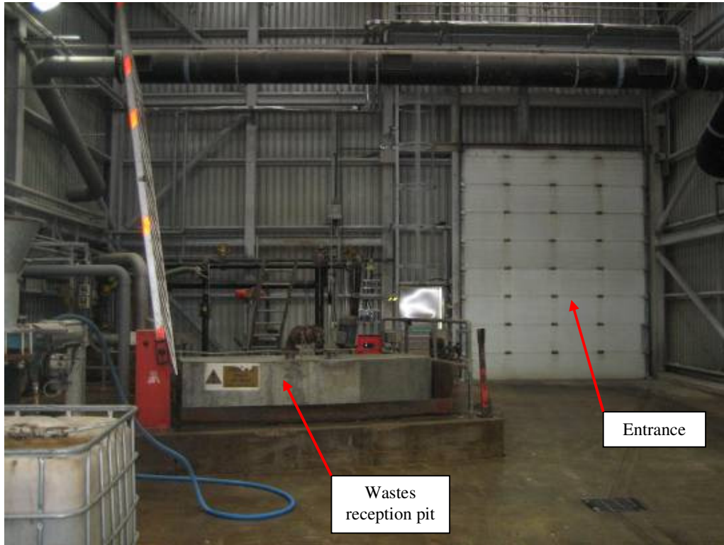
Figure 264 Wastes reception pit in enclosed wastes reception hall
