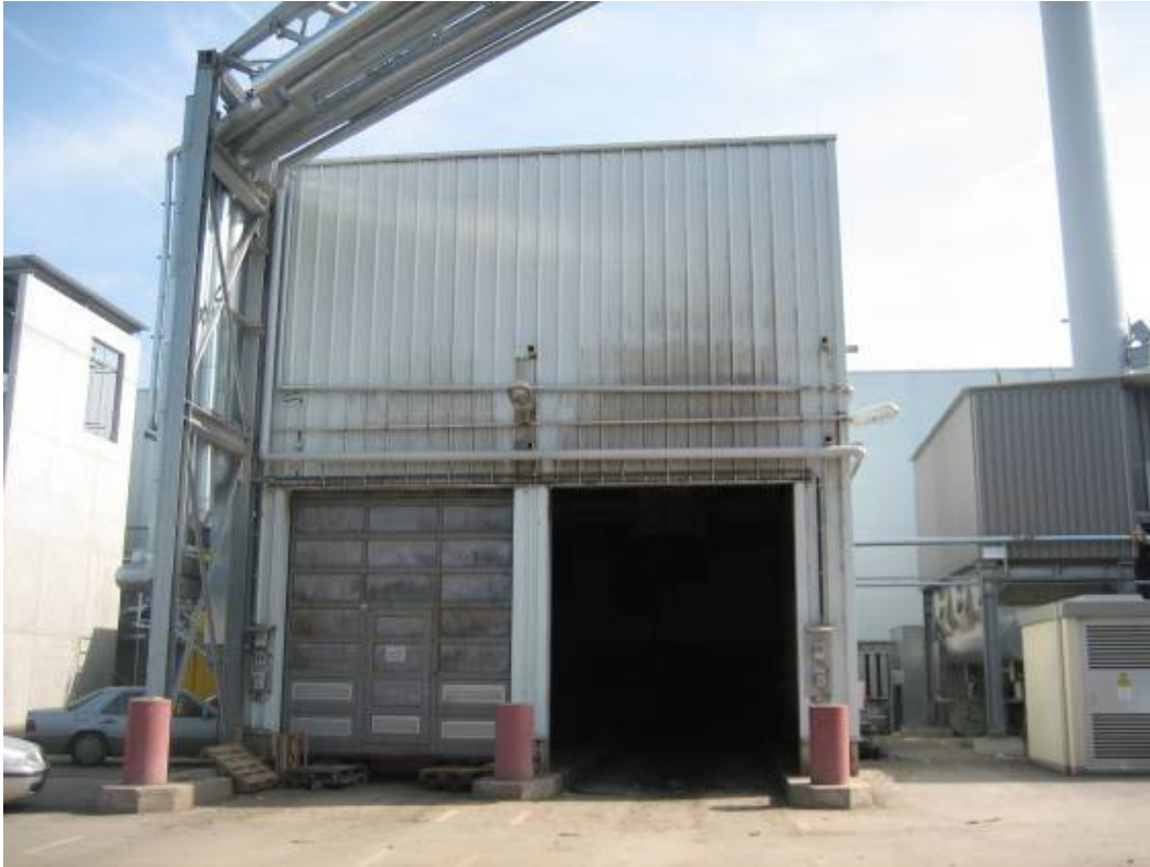
Figure 207 CLO/biostabilat loading bay at Heilbronn
