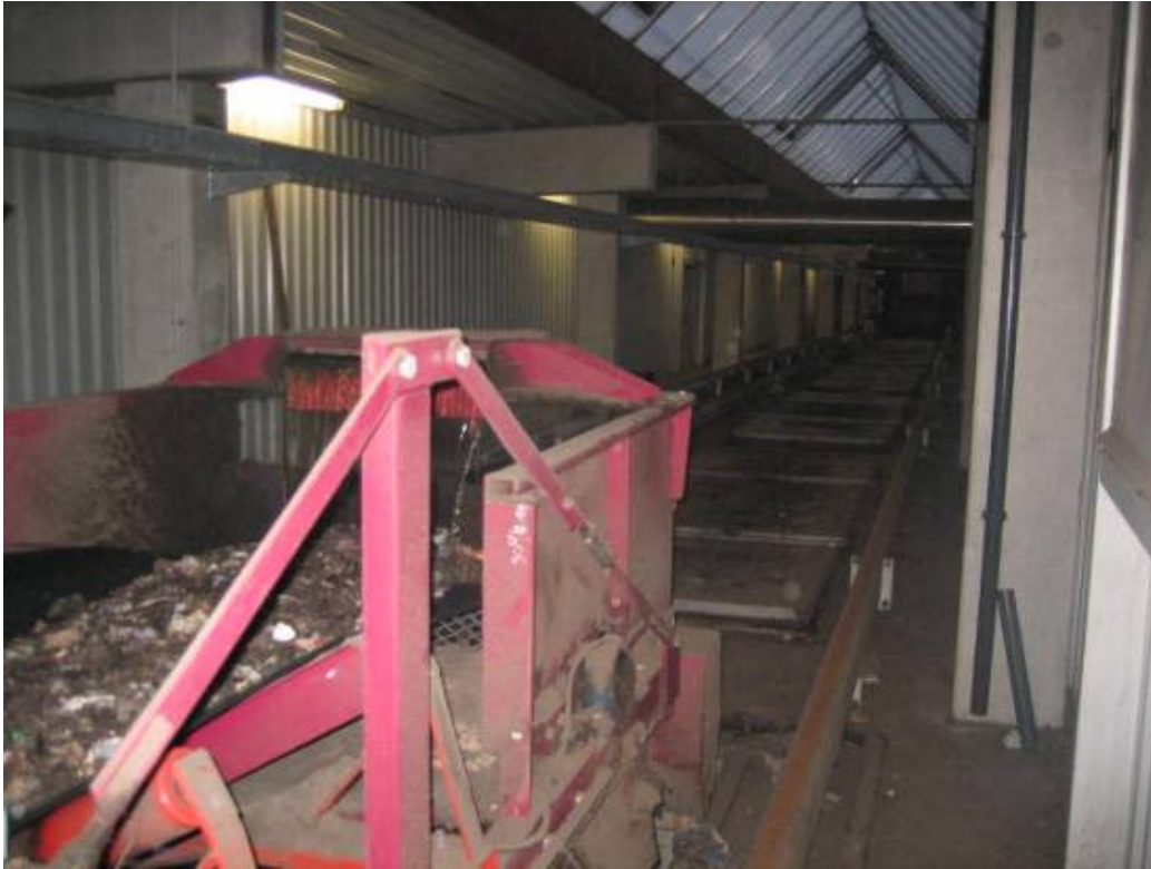
Figure 240 Waste entering tunnel composting system
