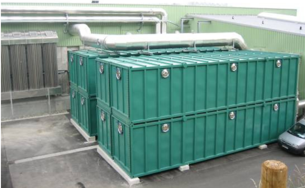
Figure 259 Biofilter for exhaust gas treatment
