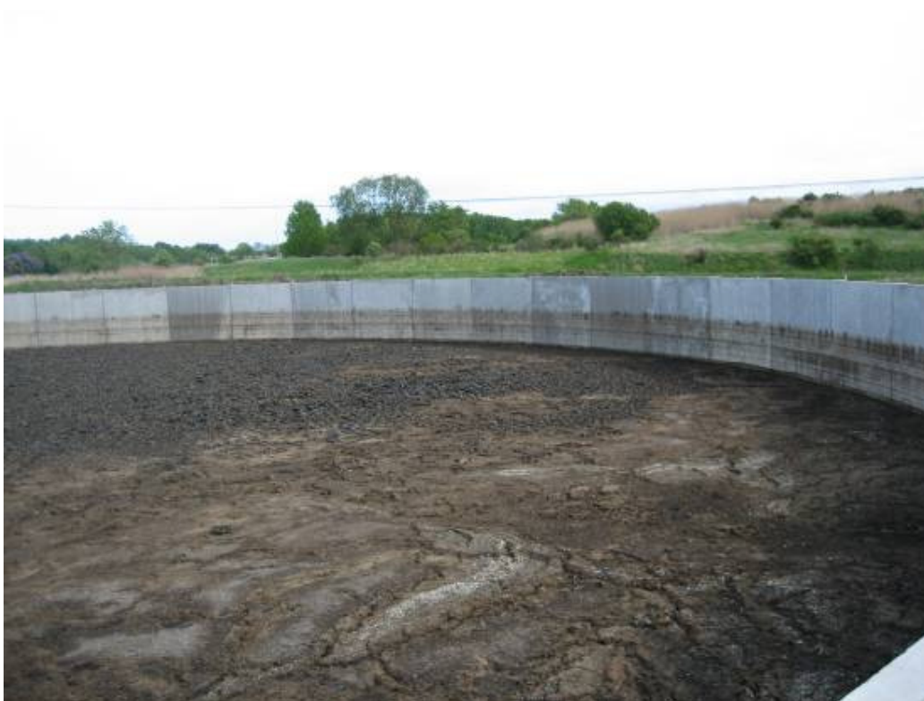
Figure 272 Inside digestate storage tank at Linköping
