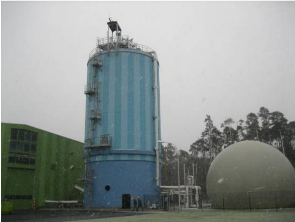
Figure 239 Dranco digester at Pohlsche-Heide
