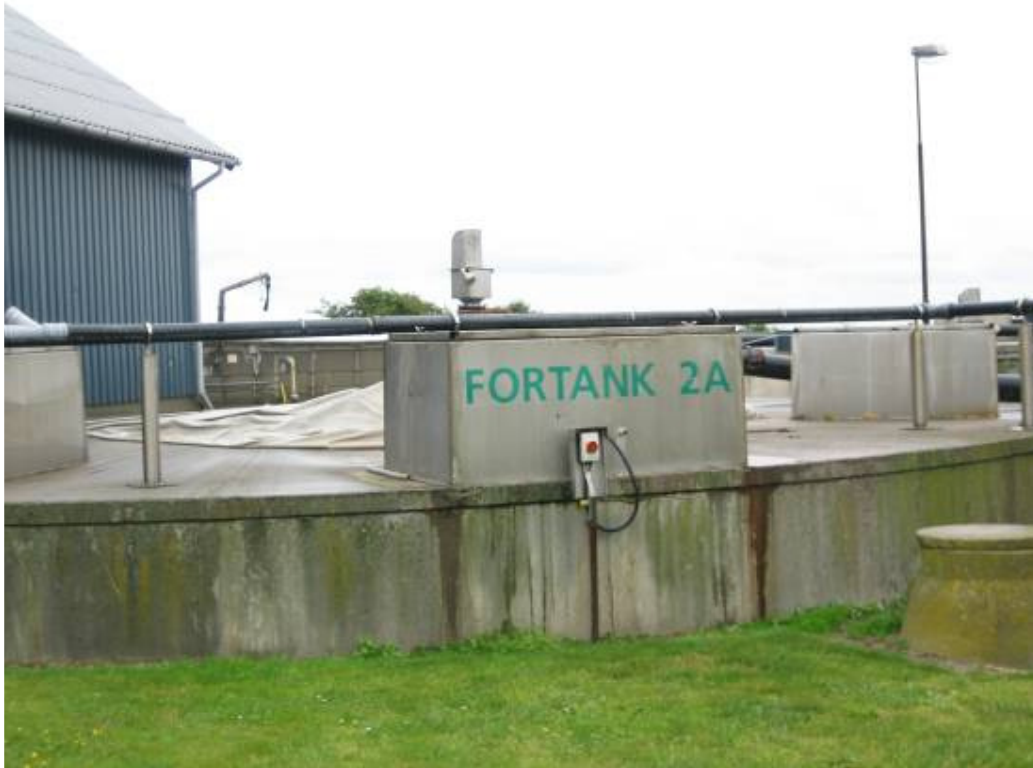
Figure 278 Wastes reception tank
