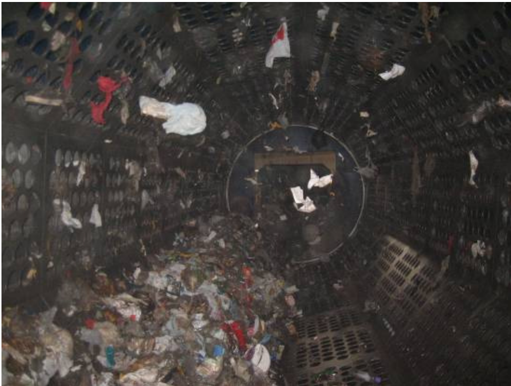
Figure 204 Inside trommel sieve at Heilbronn
