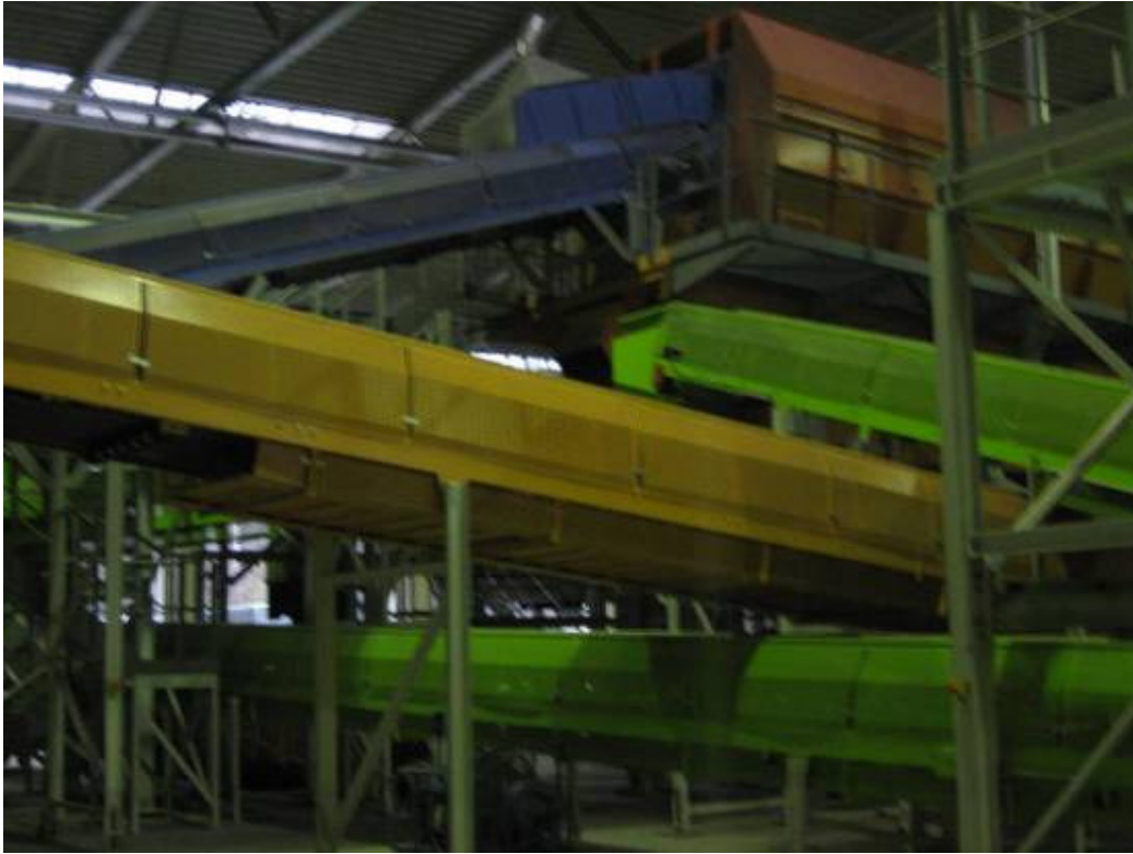
Figure 237 Conveyors between mechanical separation stages
