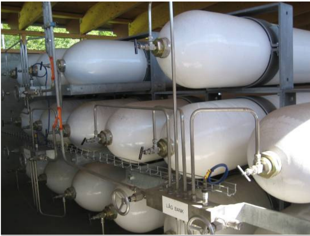
Figure 183 Biogas storage at Västerås Bus Depot
