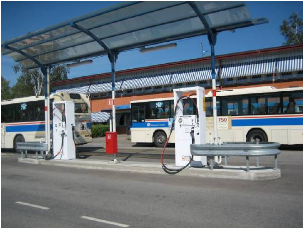
Figure 184 Biogas fuel pumps
