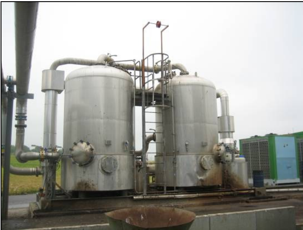
Figure 231 Gas de-sulphurisation units
