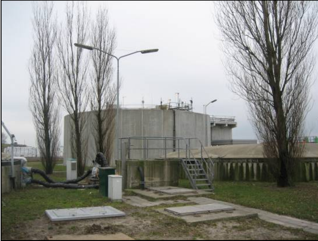
Figure 215 Wastewater treatment plant at SBI Friesland
