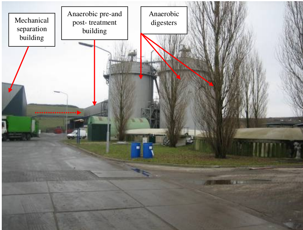
Figure 213 Anaerobic digesters at SBI Friesland
