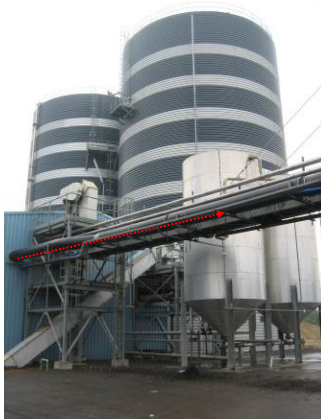
Figure 223 Anaerobic digesters
