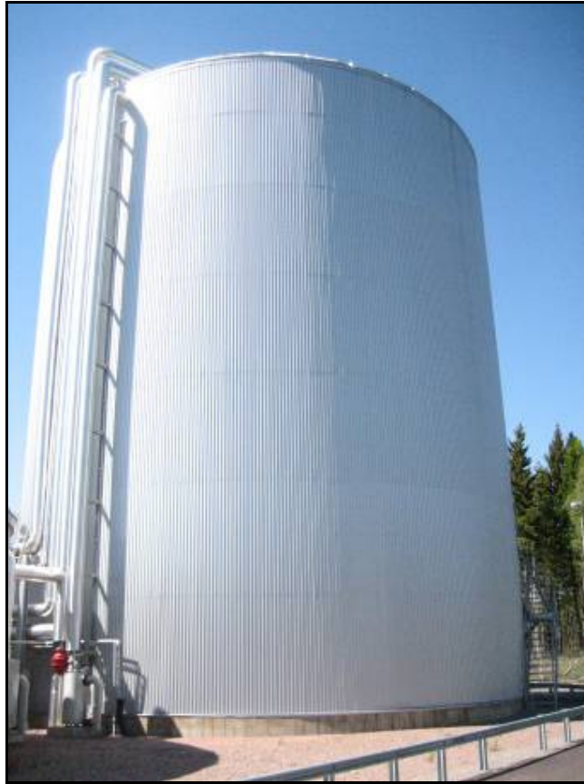
Figure 168 Anaerobic digester at Växtkraft plant
