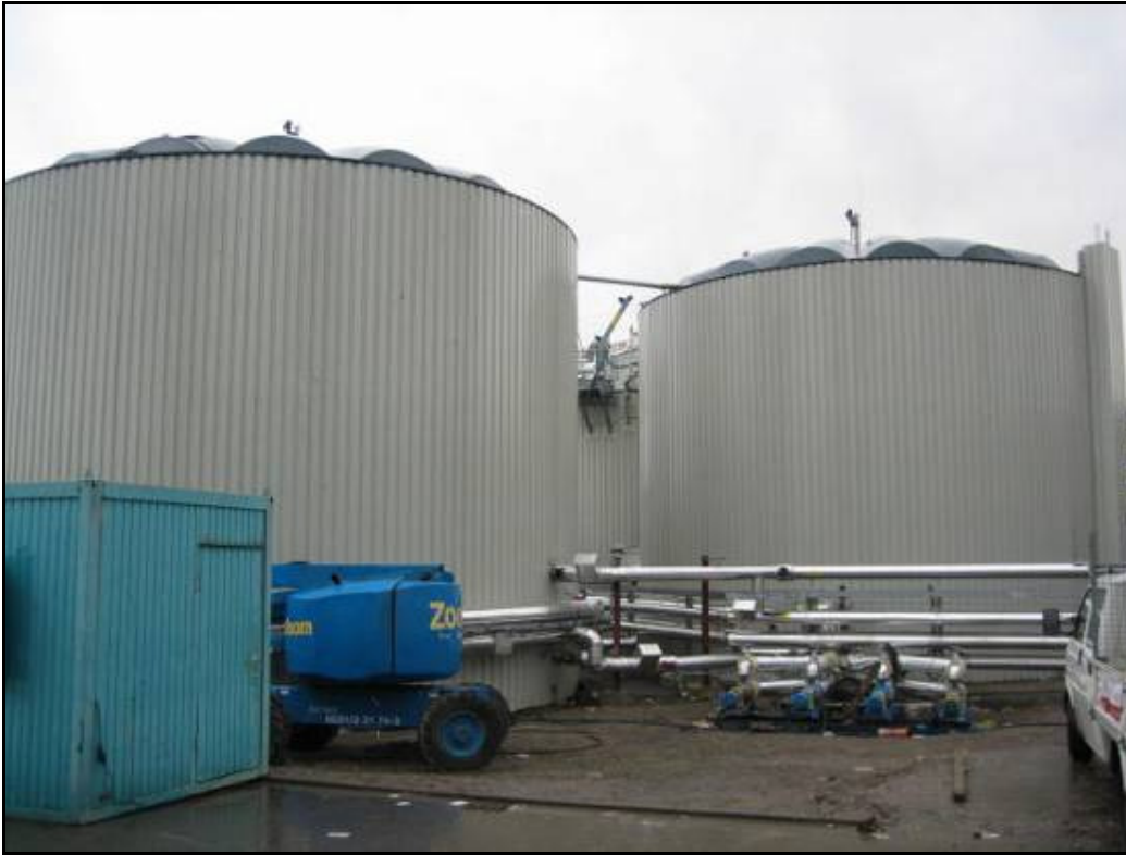
Figure 245 Hydrolysis tanks
