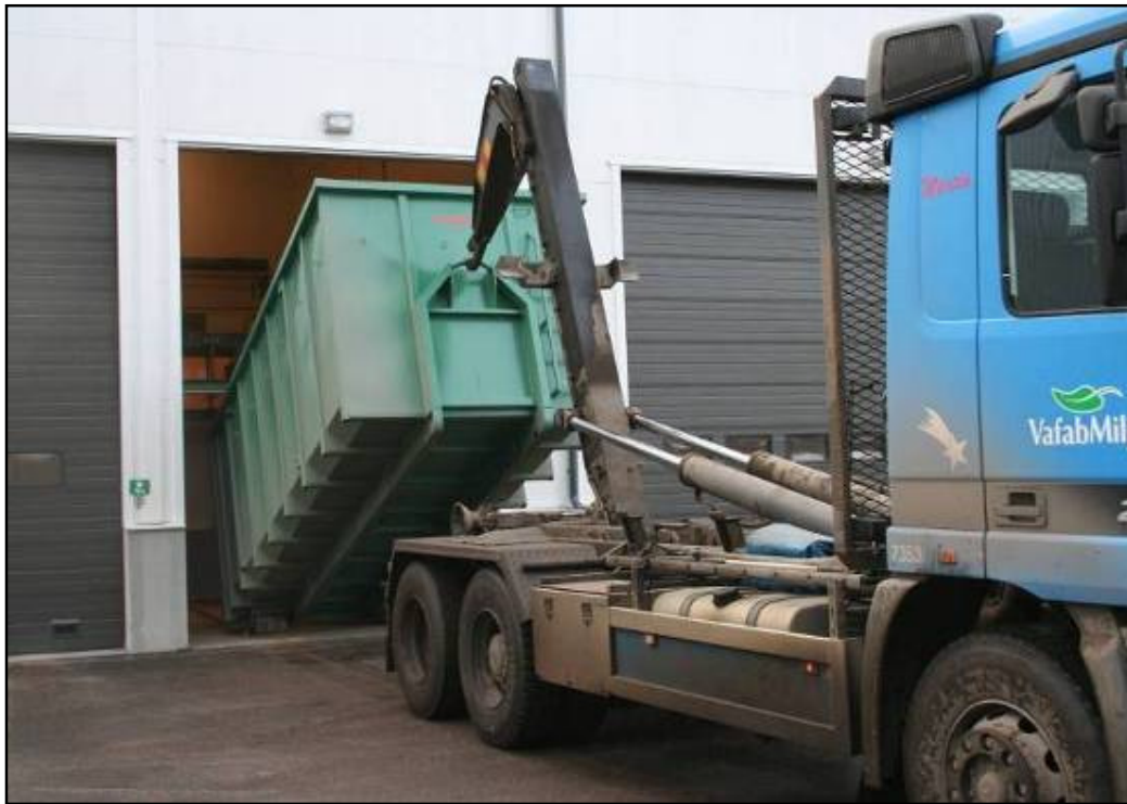
Figure 175 Truck removing solid digestate container from plant (Pettersson, 2006)
