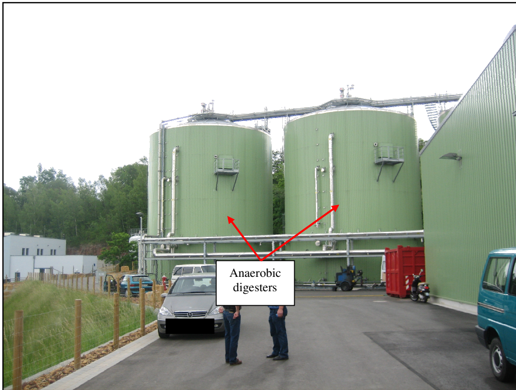
Figure 254 Two (of the three) anaerobic digesters
