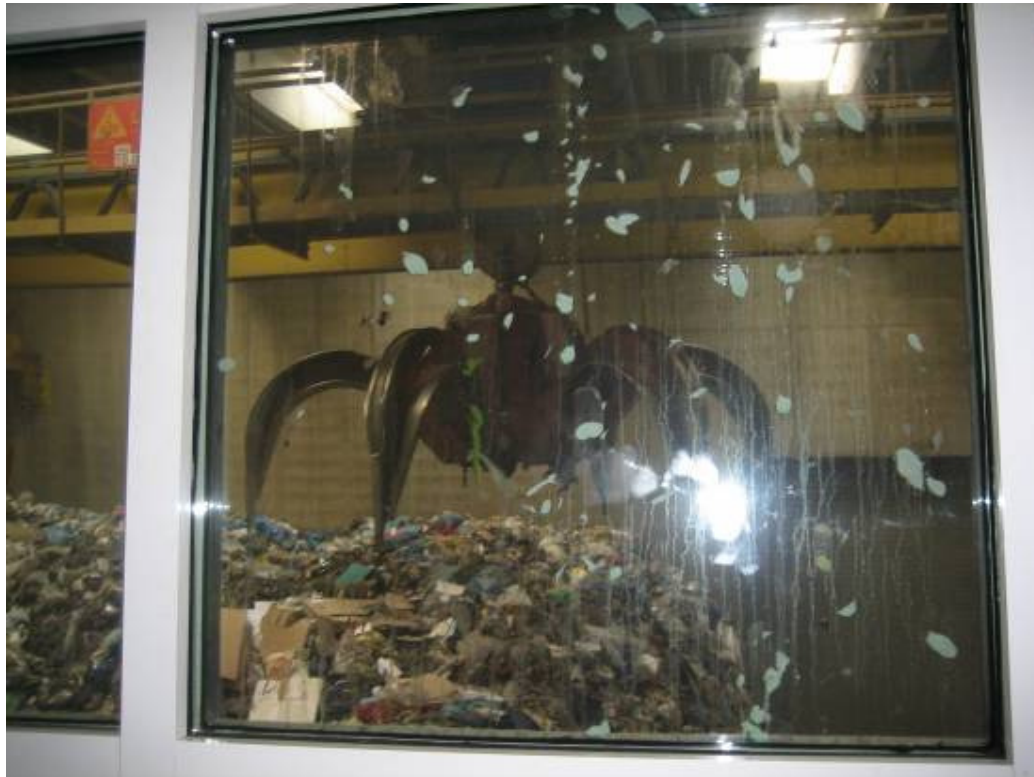
Figure 202 Wastes reception area (indoors) at Heilbronn
