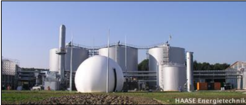
Figure 296 Luebeck MBT Plant (Haase website, accessed July 2006)
