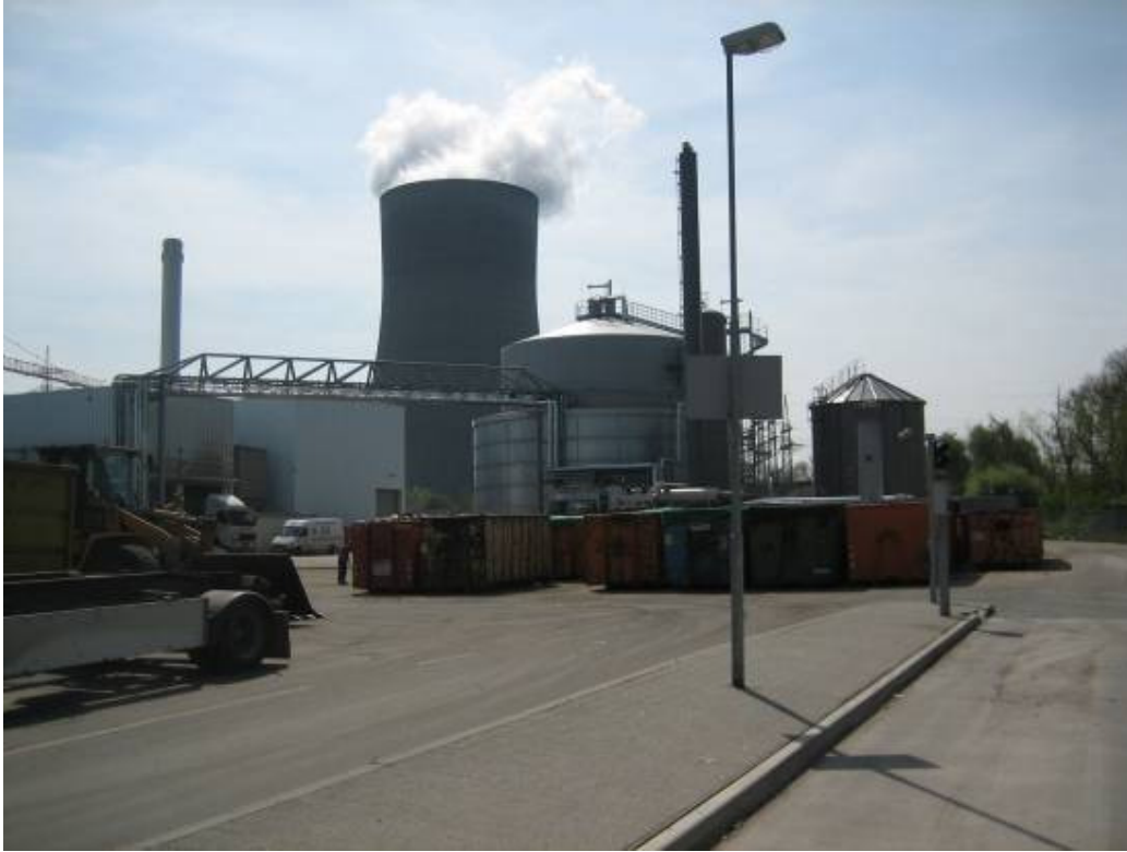
Figure 209 ISKA Plant at Heilbronn (power station in background)
