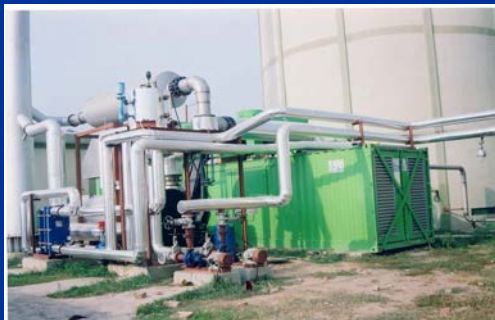
GAS ENGINE AND WASTE HEAT RECOVERY UNIT
