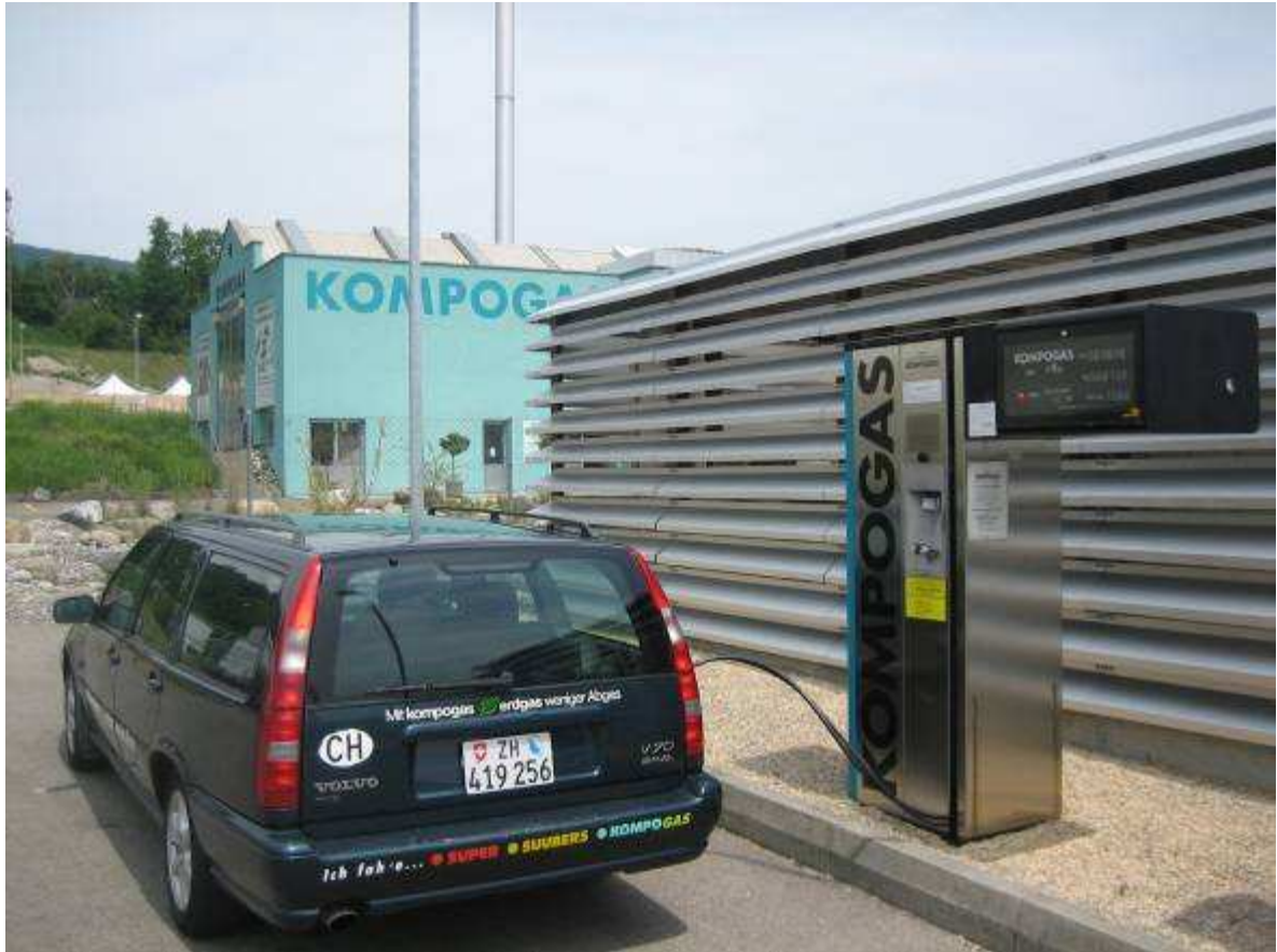
Figure 10 Biogas filling station at Otelfingen
