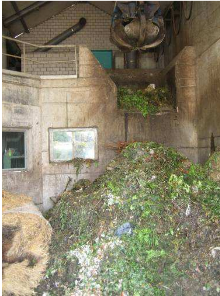
Figure 5 Wastes reception pit and picking crane
