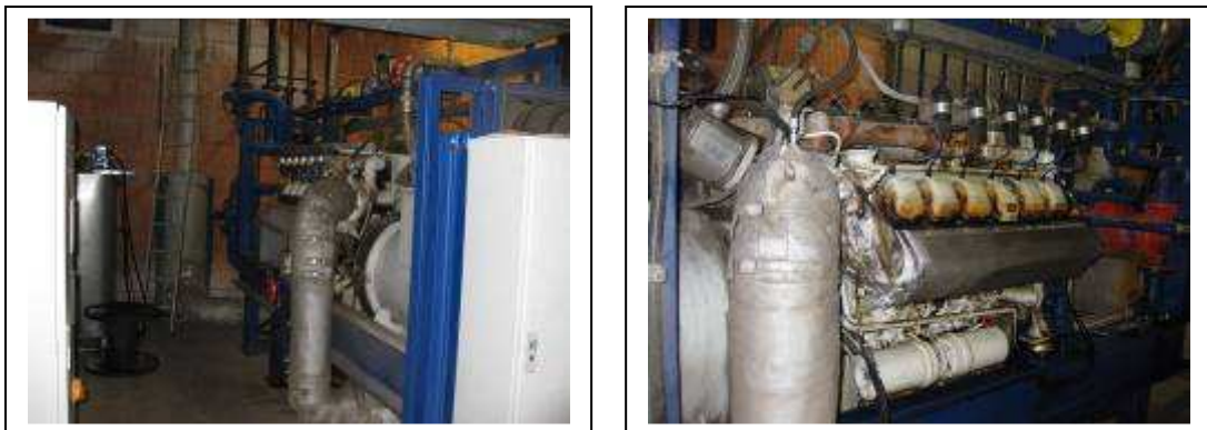
Figures 22 and 23 – CHP engines used at the energy crop plant
