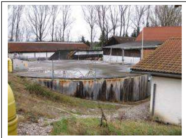
Figure 8 – Secondary Digester
