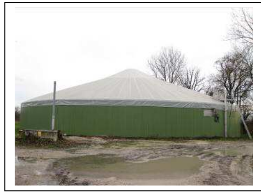
Figure 12 – Digestate storage tank with flexible membrane roof and mechanical mixing
